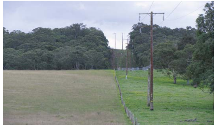
Image: Existing Kurri to Stroud Road powerline
