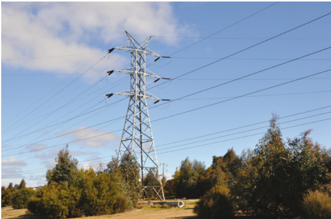
Above: The existing 132 kV steel structure is being dismantled in the coming months to make way for new concrete poles similar to the sample pole shown in the above image to the right.
