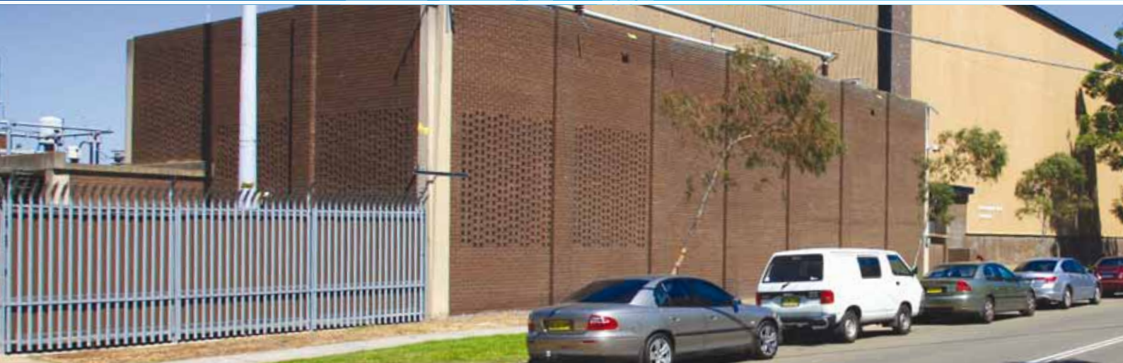
The existing Beaconsfield West substation will be redeveloped over four years with construction expected to be completed by the end of 2012.
