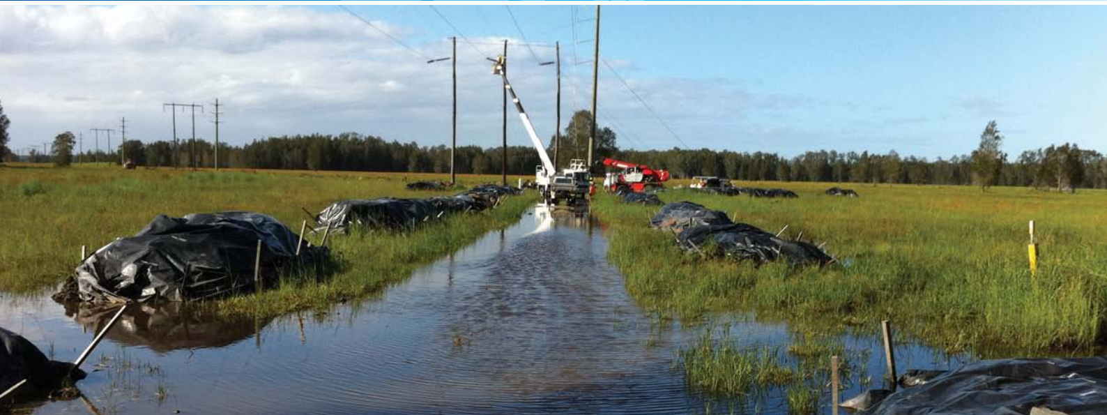
TransGrid contractor PowerServe works to deliver the project in difficult conditions.
