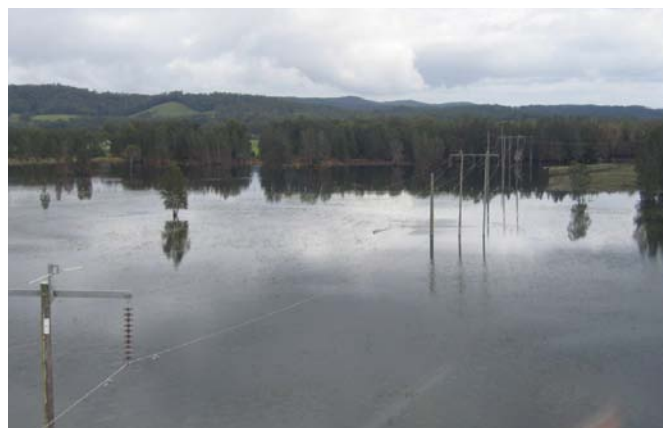
Rain and flooding has caused significant delays to the Kempsey to Port Macquarie Project.
