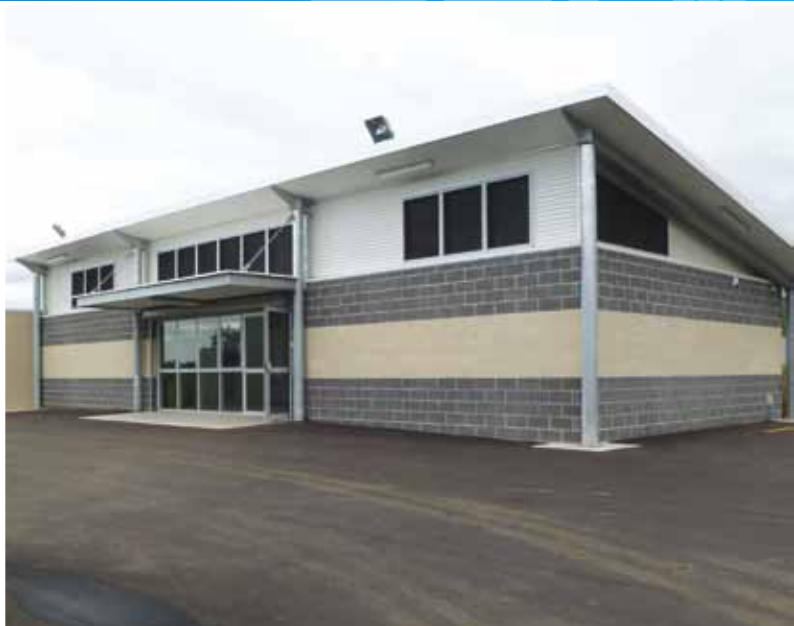
TransGrid constructed the new Rifle Range and Pigeon Club next to the site of the future Holroyd Substation.
