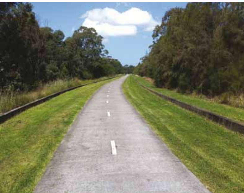
TransGrid is proposing to bury the electricity cables beside the canal reserve cycleway between a section of Hyland Road and Palmer Street at Guildford.
