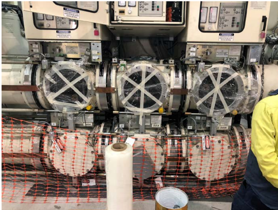
Figure 1: Parawebbing used to barrier out in service apparatus from accessible apparatus for GIS. Accessible gas points identified with yellow caps
