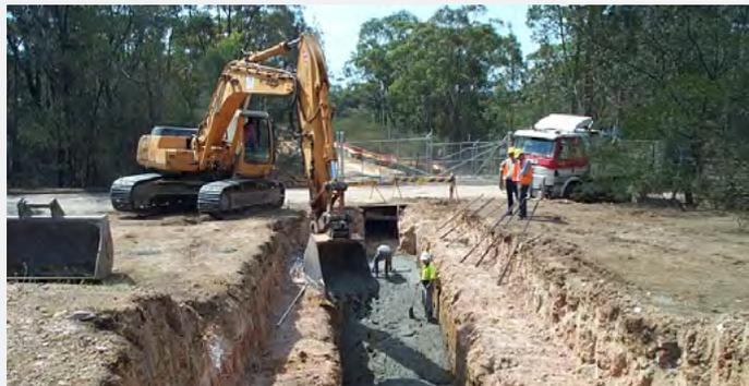
TransGrid site representative. Where heavy 'crawler' or 'vibration' machinery are to operate above the cables, a minimum cover of 900mm to the cables is required. Where this cover is unachievable, TransGrid may require the use of heavy steel plates to distribute the load.
