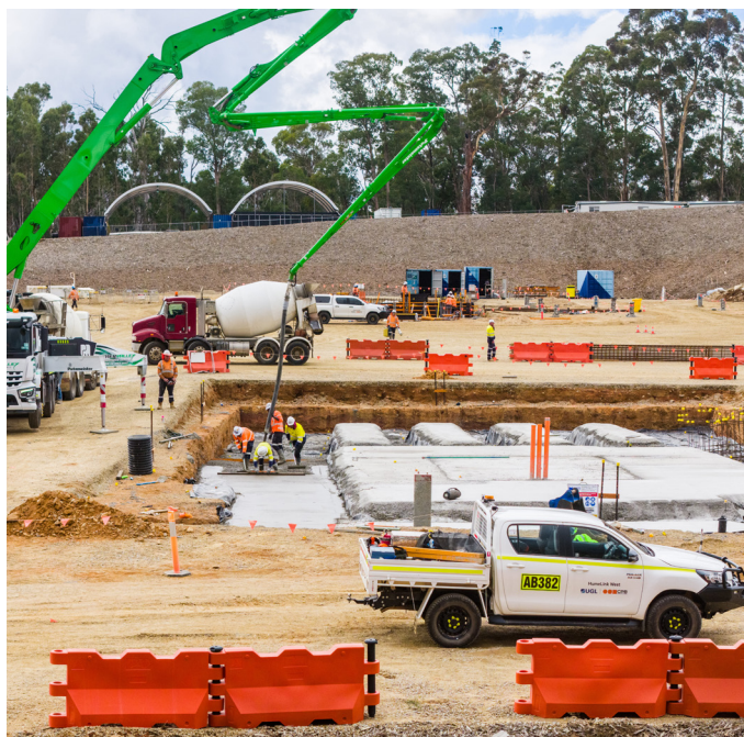
Concrete from the new batch plant is poured at Maragle Substation.
