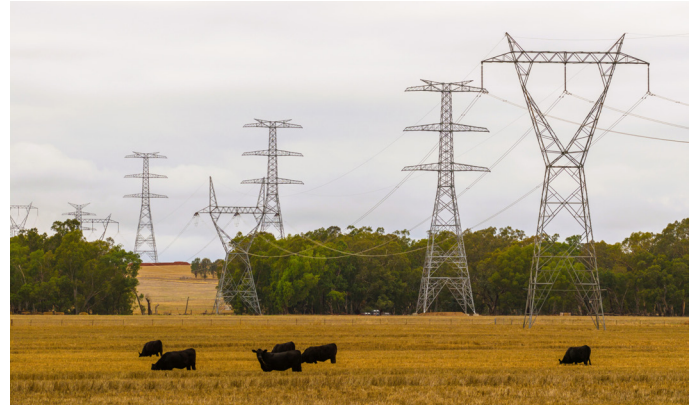
New transmission towers erected near the new Gugaa Substation.
