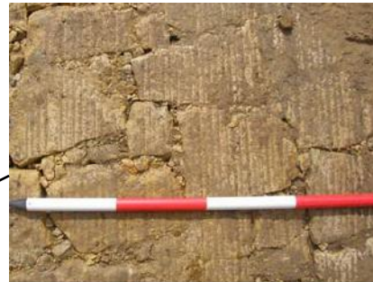
Figure 2: Close up detail of the sandstone surface showing material type, formation and construction detail. This is essential for establishing date of the feature.
