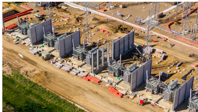
Transformers being installed and tested at Gugaa Substation recently.
