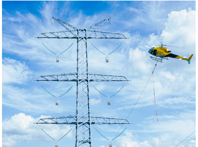
Recent helicopter conductor stringing on HumeLink East.
