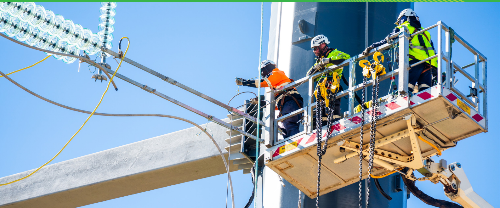
Workers install conductors on three new monopoles that connect an existing transmission line with HumeLink at Gregadoo.
