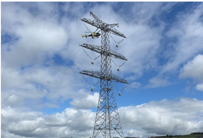
Helicopter stringing underway near Dalton
