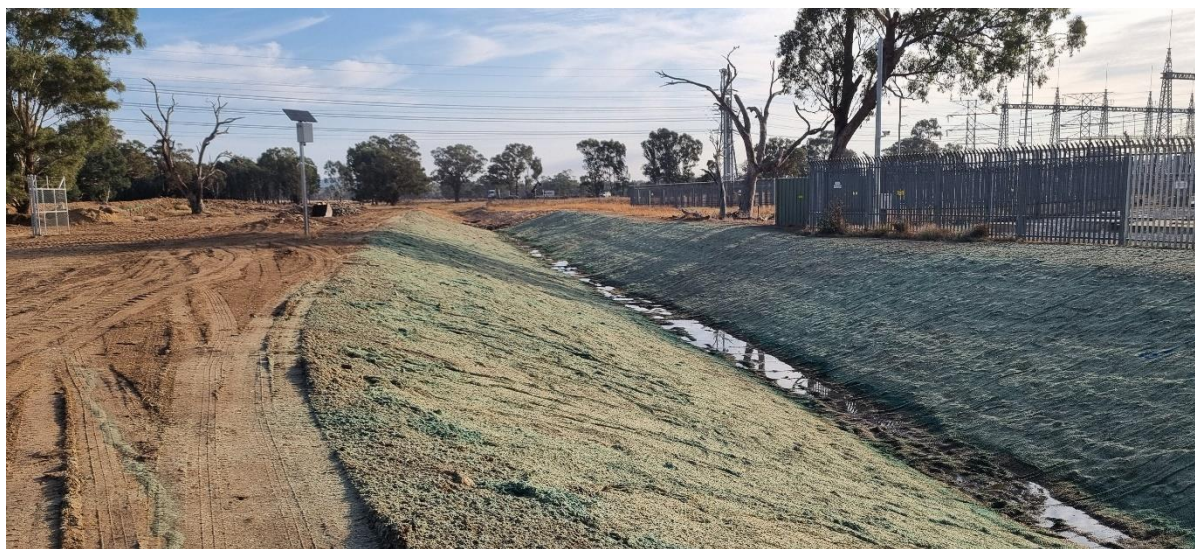
Photograph 2 – Drain stabilisation at Wagga Wagga substation.
