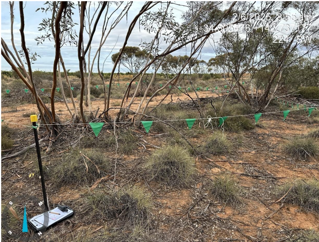
Photograph D.1 Thyme Rice-flower special biodiversity protection zone to delineate areas of avoidance during clearing (L2, Tower 661)
