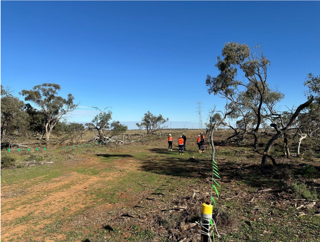
Photograph D.17 Partial clearing, showing centreline (Clearance Area A) delineated by flagging. B4 and B10 clearing zones with retained vegetation are beyond the flagging (Line 2, Tower 180)
