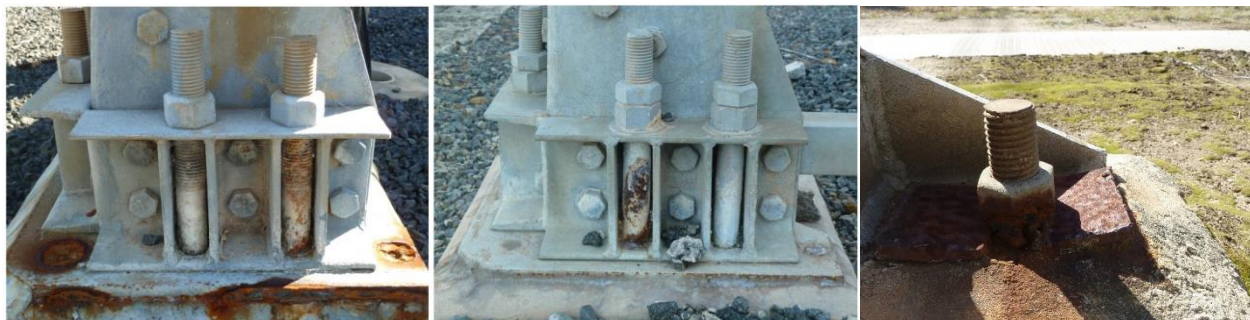
Figure 2-4 Typical corrosion to holding down bolts and baseplates
