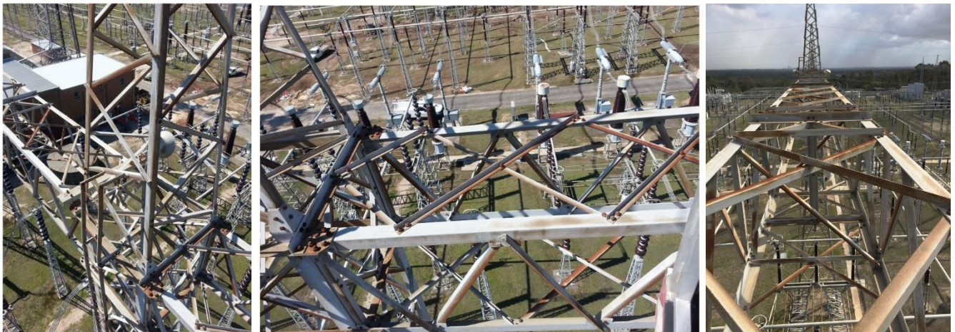
Figure 2-3 Typical gantry steel members showing corrosion
