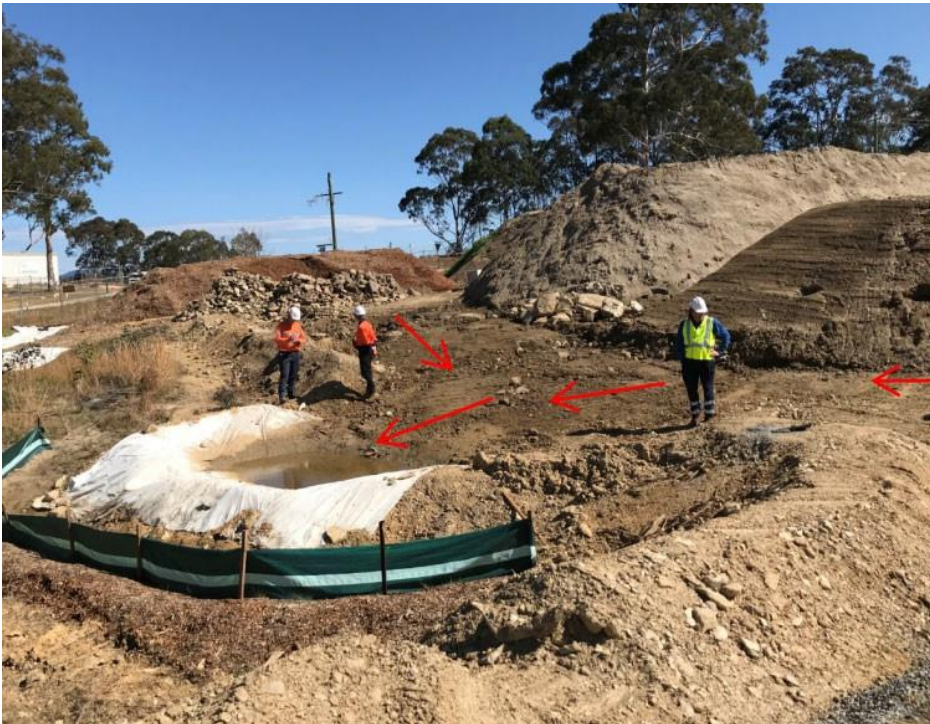
Picture 5 Downslope controls
