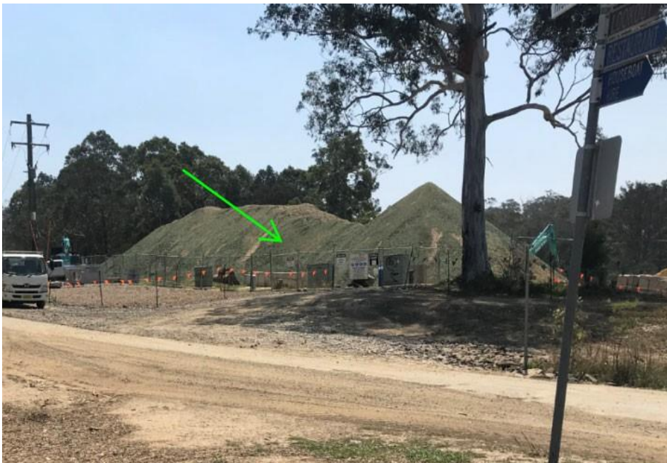
Picture 8 Soil Binder Application
