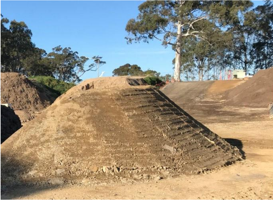
Picture 1 Bucket pressed stockpile
