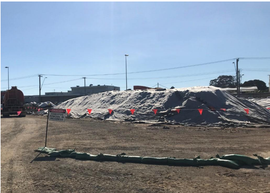
Picture 2 Asbestos stockpile (Unexpected find)
