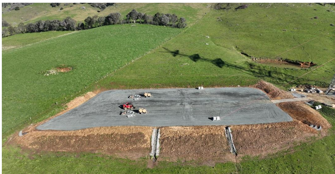
An example brake and winch pad near Tumut.
