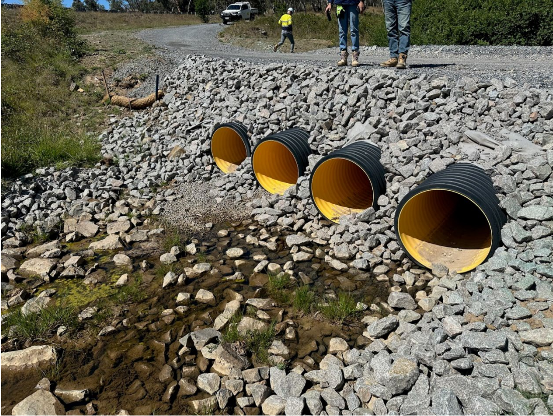
Photo 60: Culvert creek crossing
