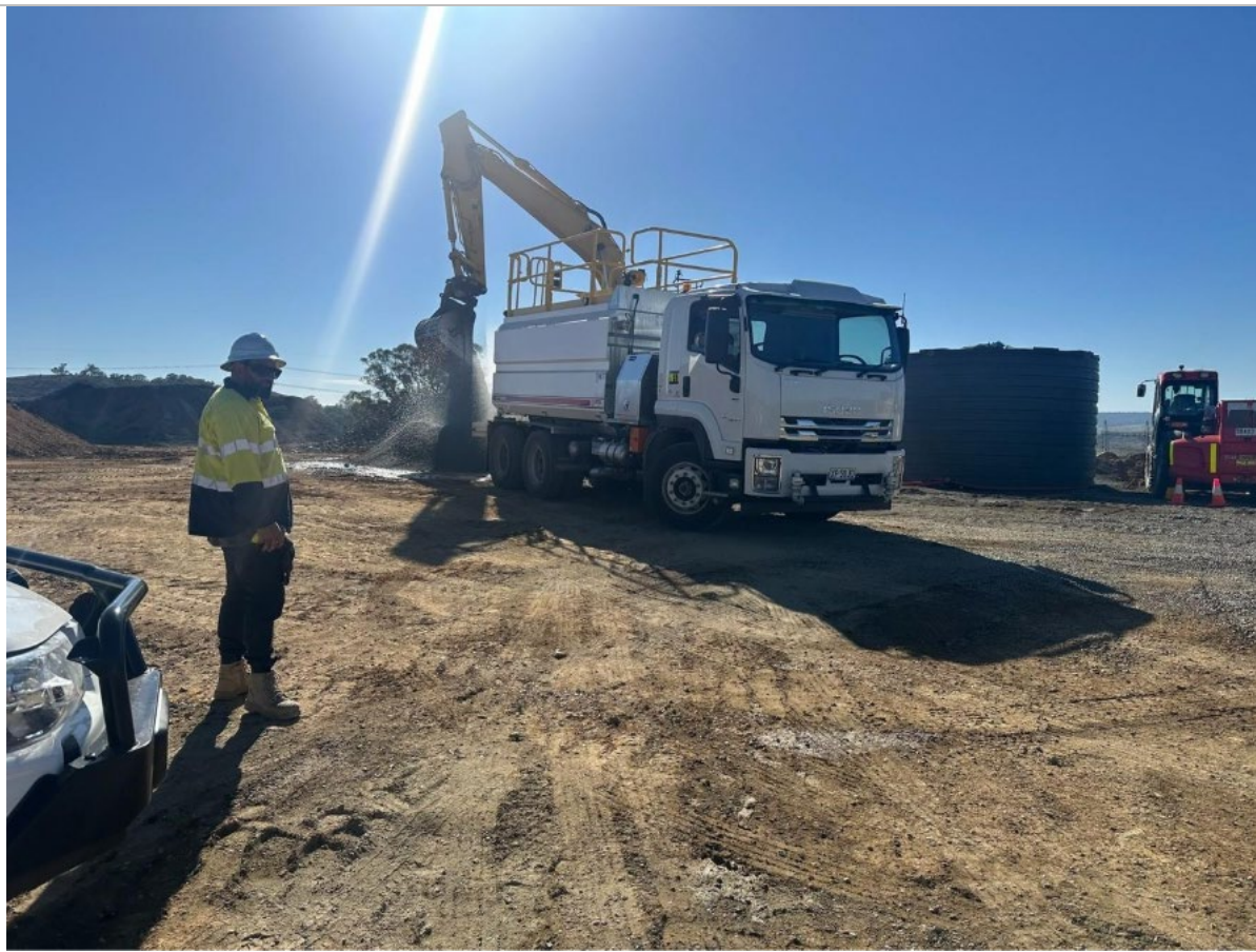
Photo 41: Stockpile watering for dust suppression
