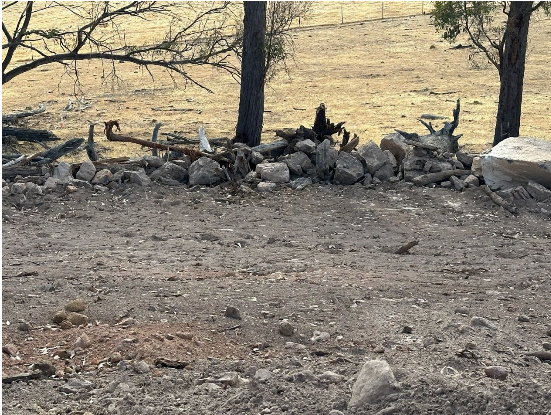
Photo 58: Rock sediment check bund
