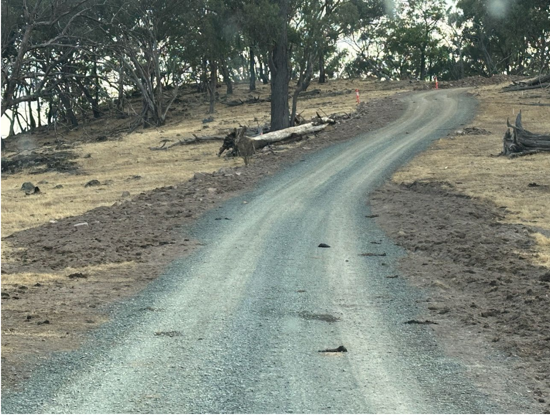
Photo 50: Graded access and topsoil preserved for rehabilitation
