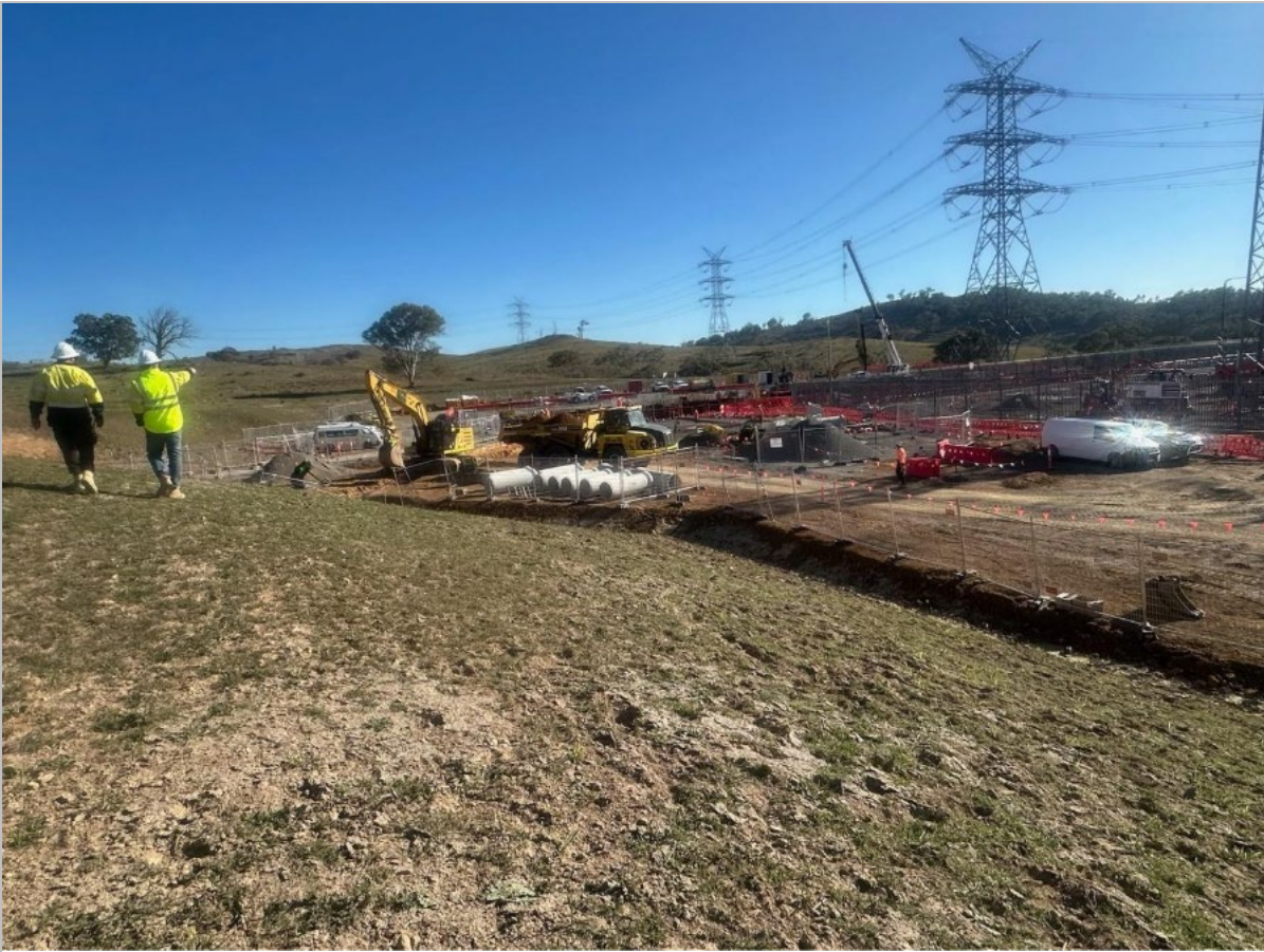
Photo 35: General construction and embankment rehabilitation
