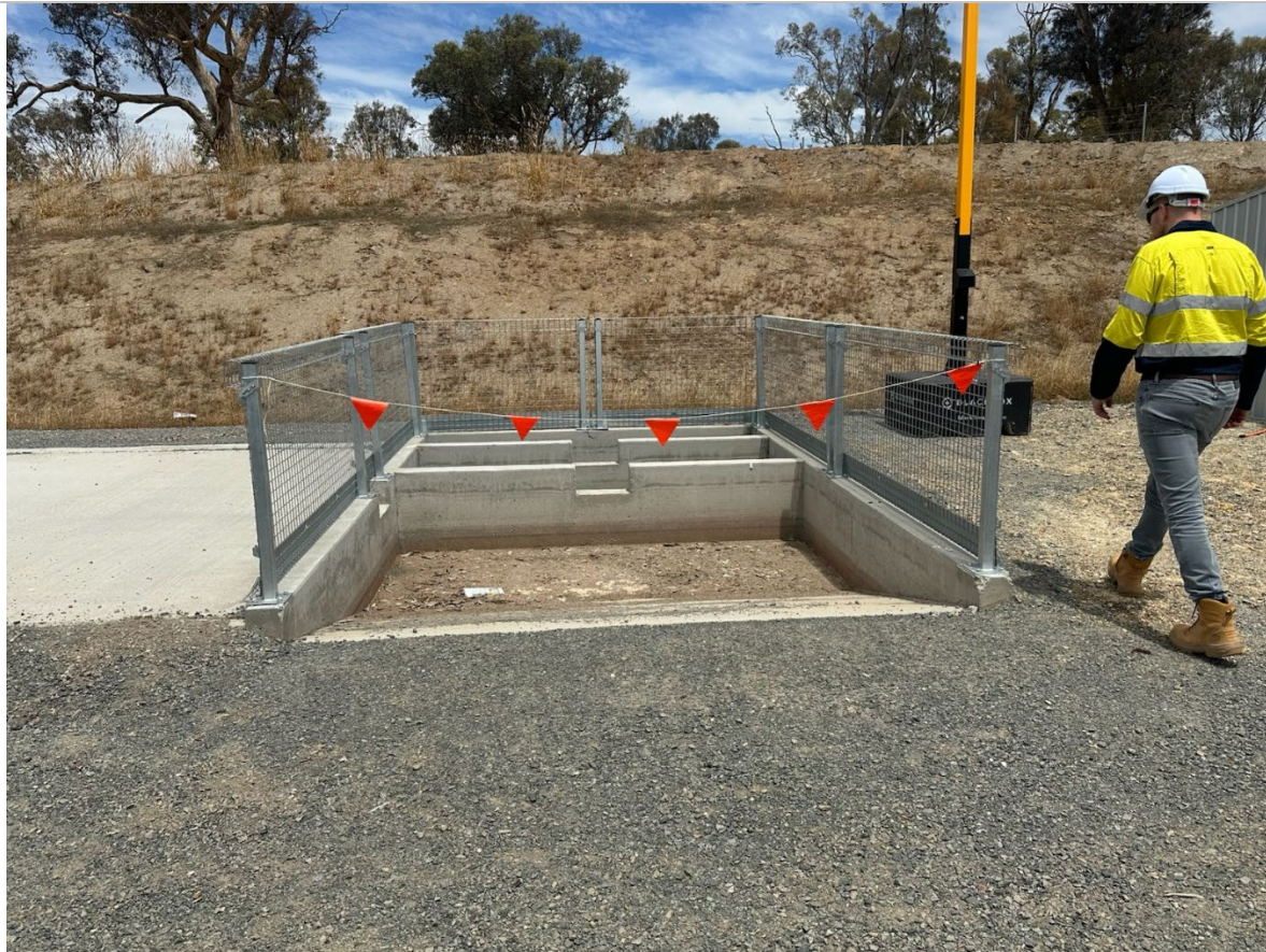
Photo 21: Bunded concrete washout area
