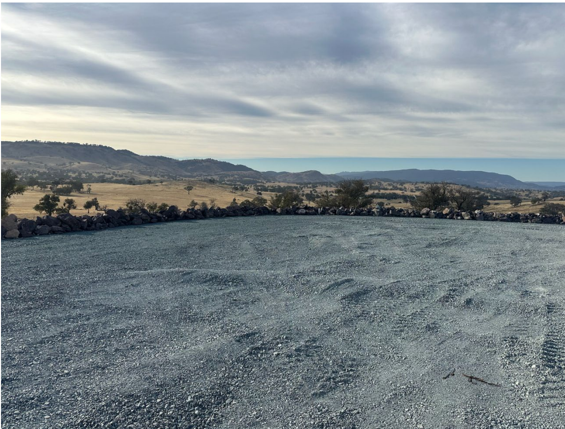
Photo 51: Stabilised construction PAD ready for piling contractor
