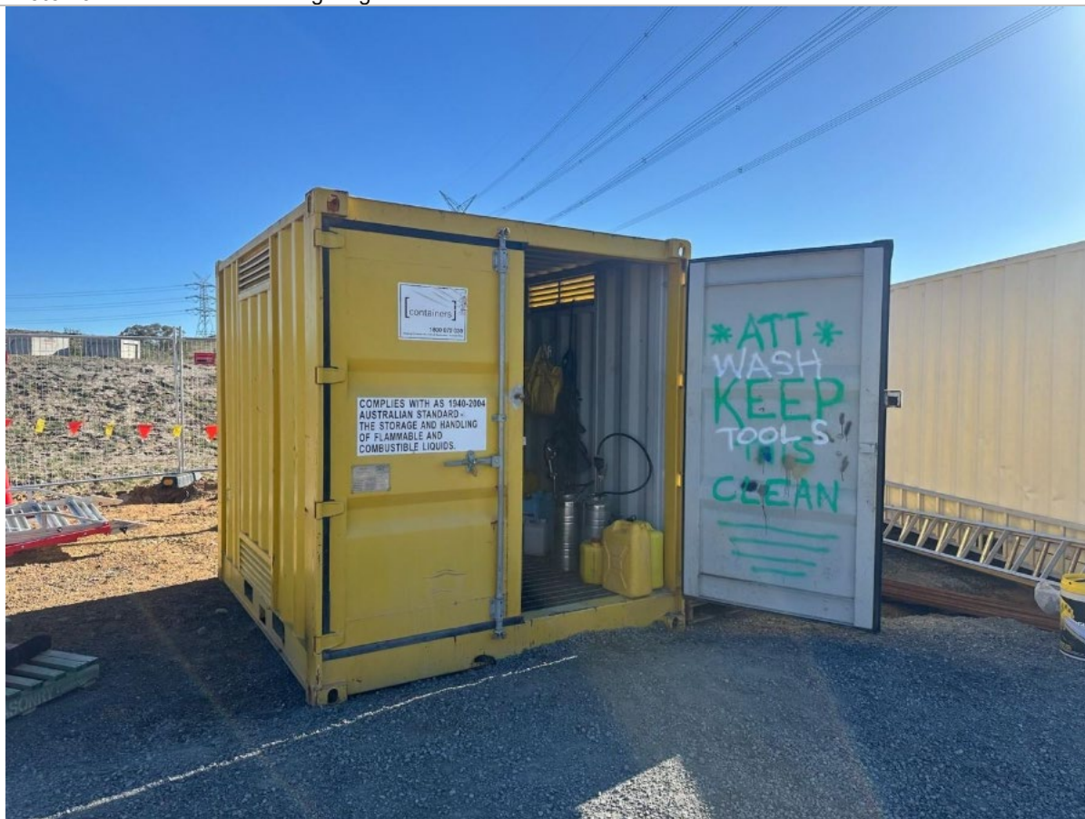
Photo 44: Chemical storage container
