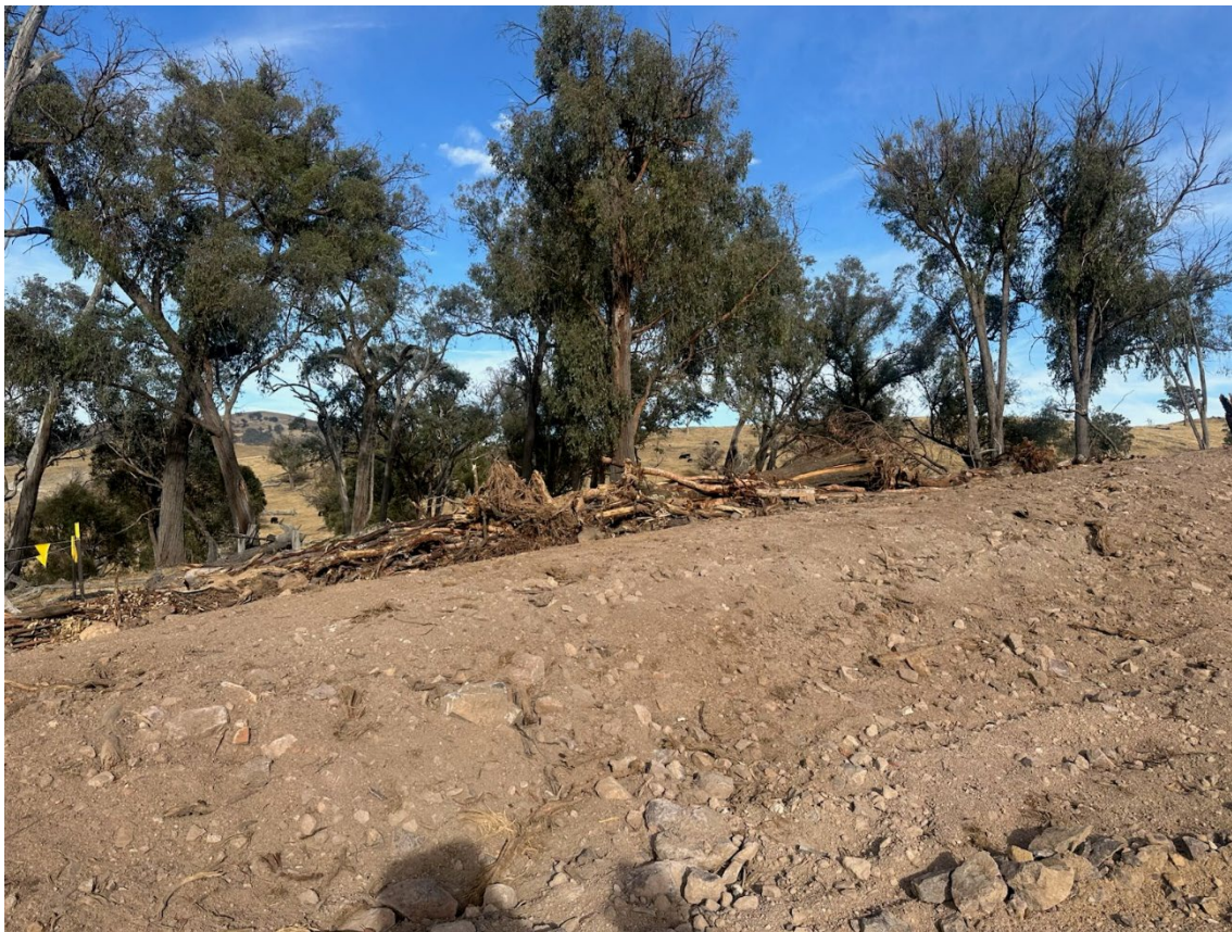
Photo 65: Retained timber for habitat reuse and sediment control
