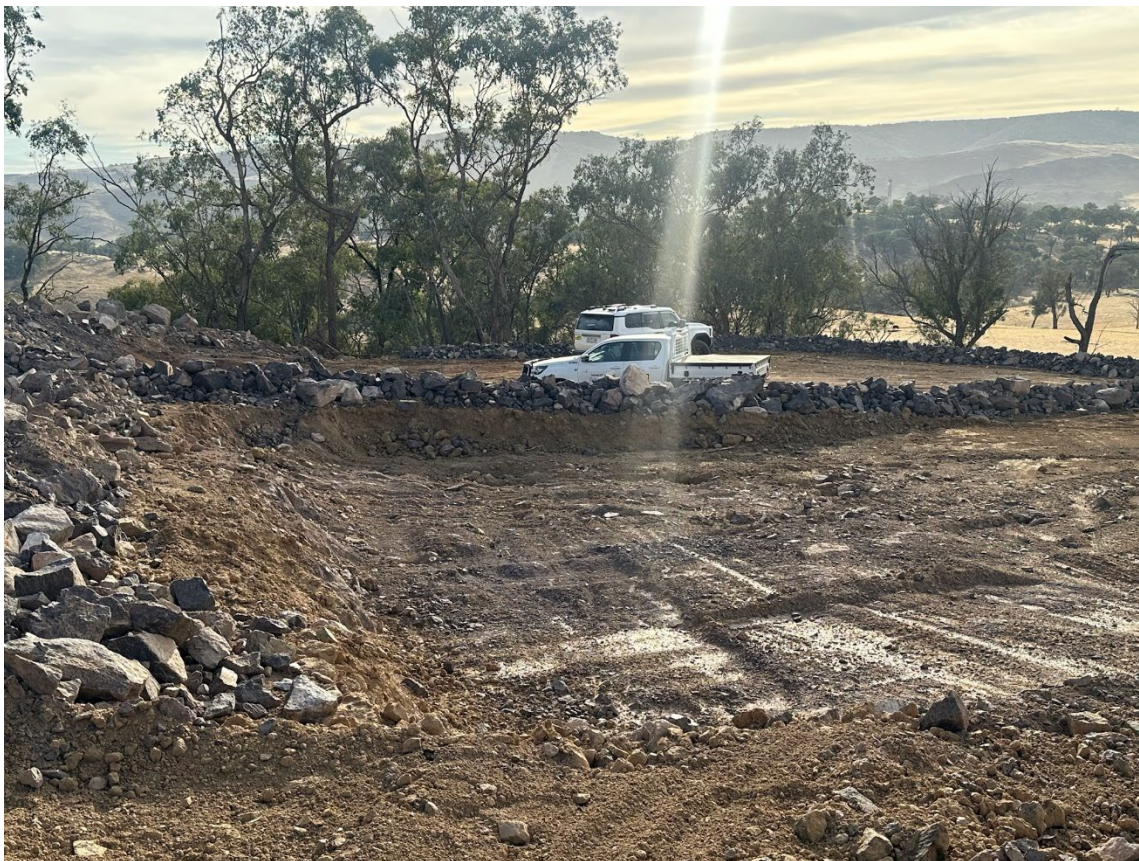
Photo 57: Tower PAD excavation and rock sediment bunds
