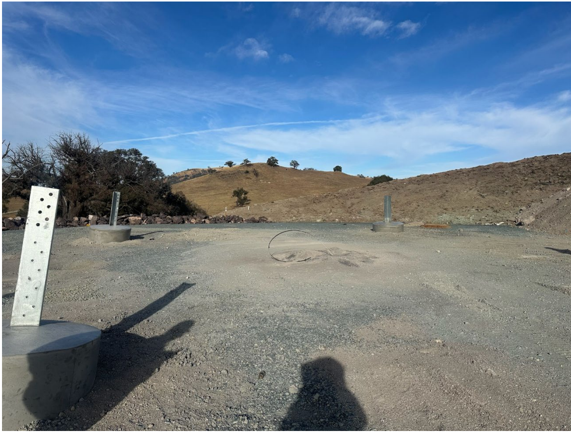
Photo 52: Tower base installation
