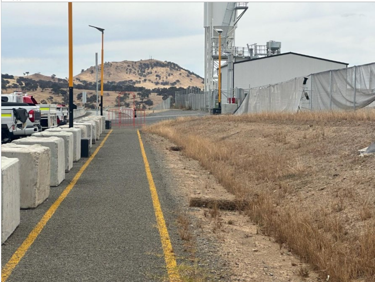
Photo 8: Internal drainage and stabilised batter
