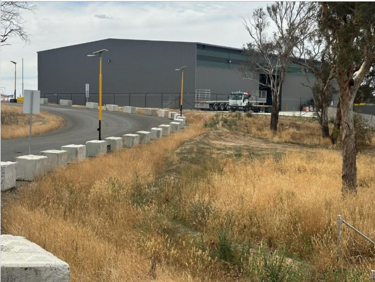
Photo 6: Site drainage and rehabilitation
