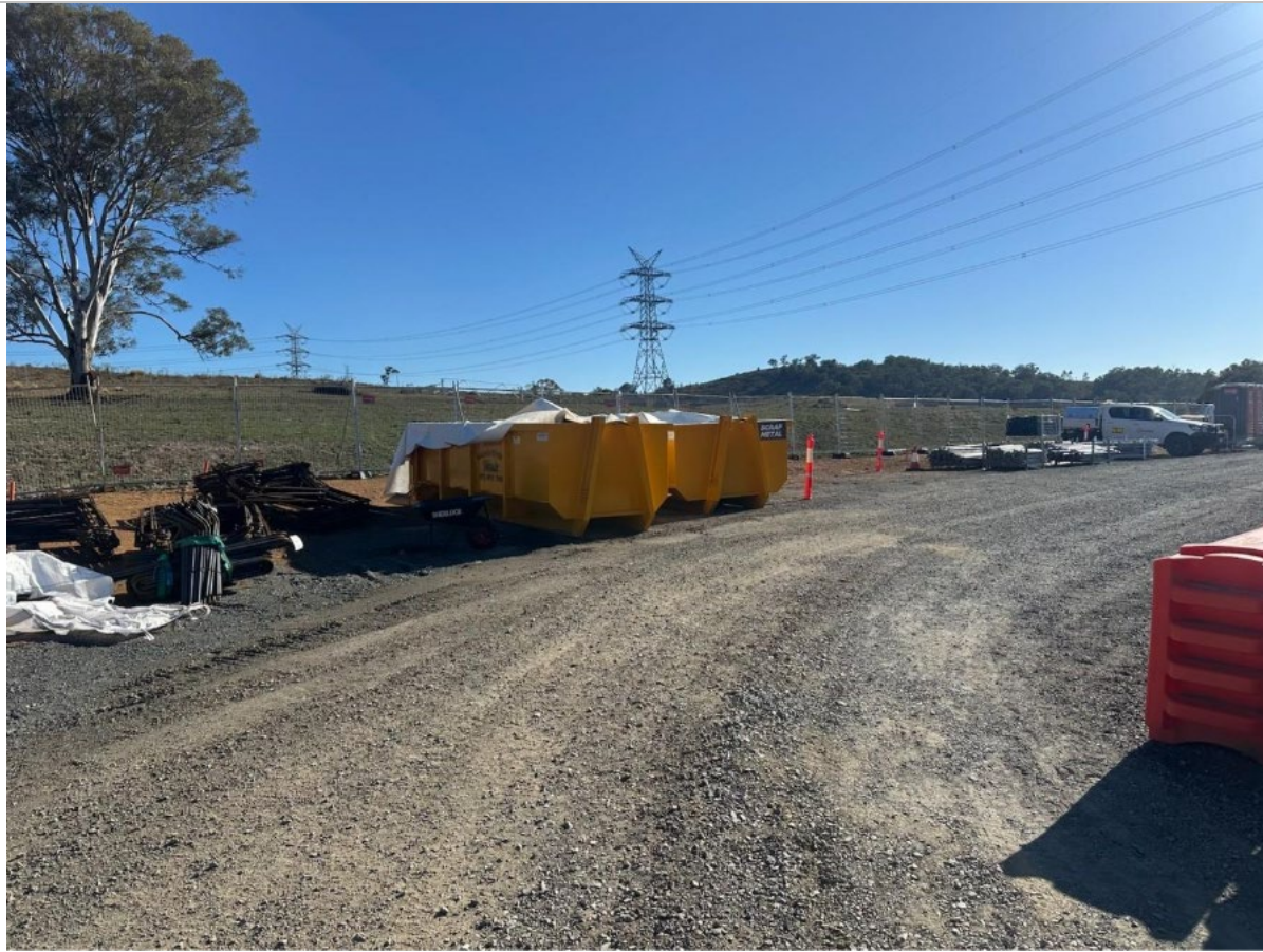
Photo 45: Waste and recycling skip bins
