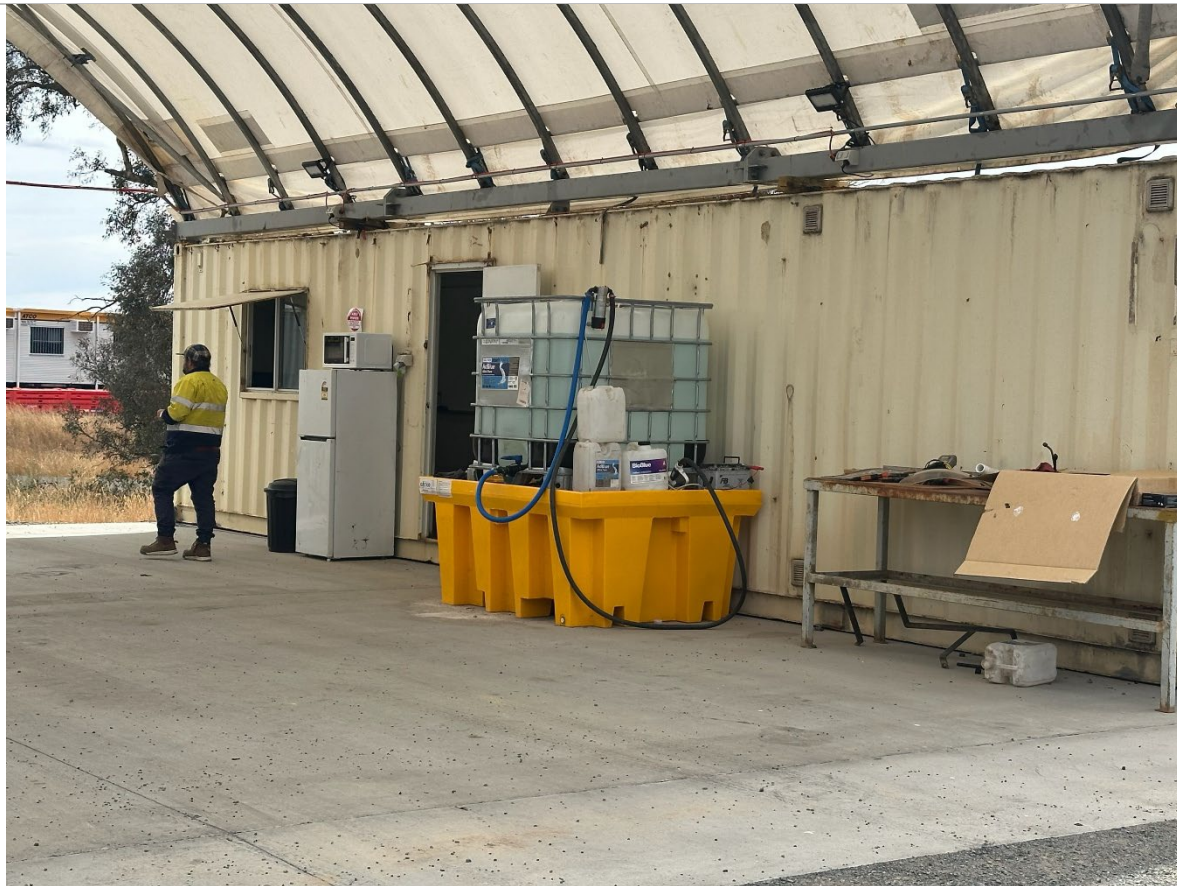
Photo 22: Chemical containment bunding
