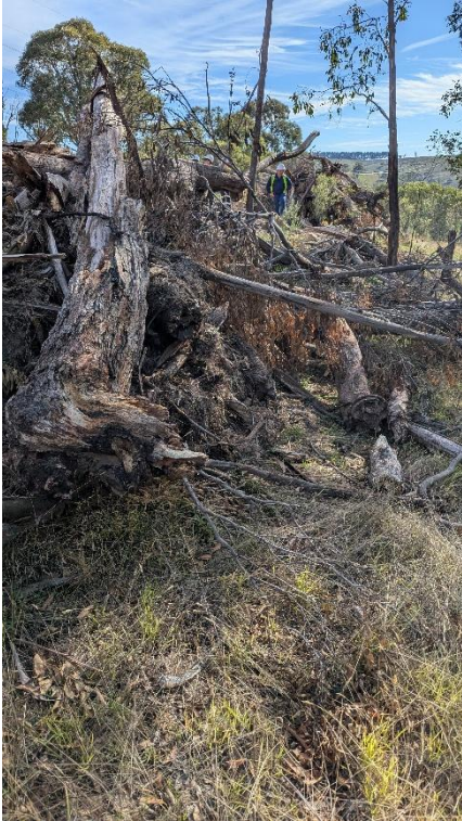
Photo 9: Coarse woody debris used to control sediment dispersal below the tower pad at Tower 55 on BY-030, showing sediment not extending beyond the control measure
