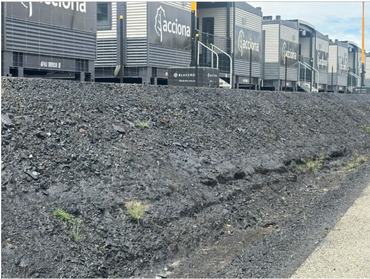
Photo 7: Stabilised batter
