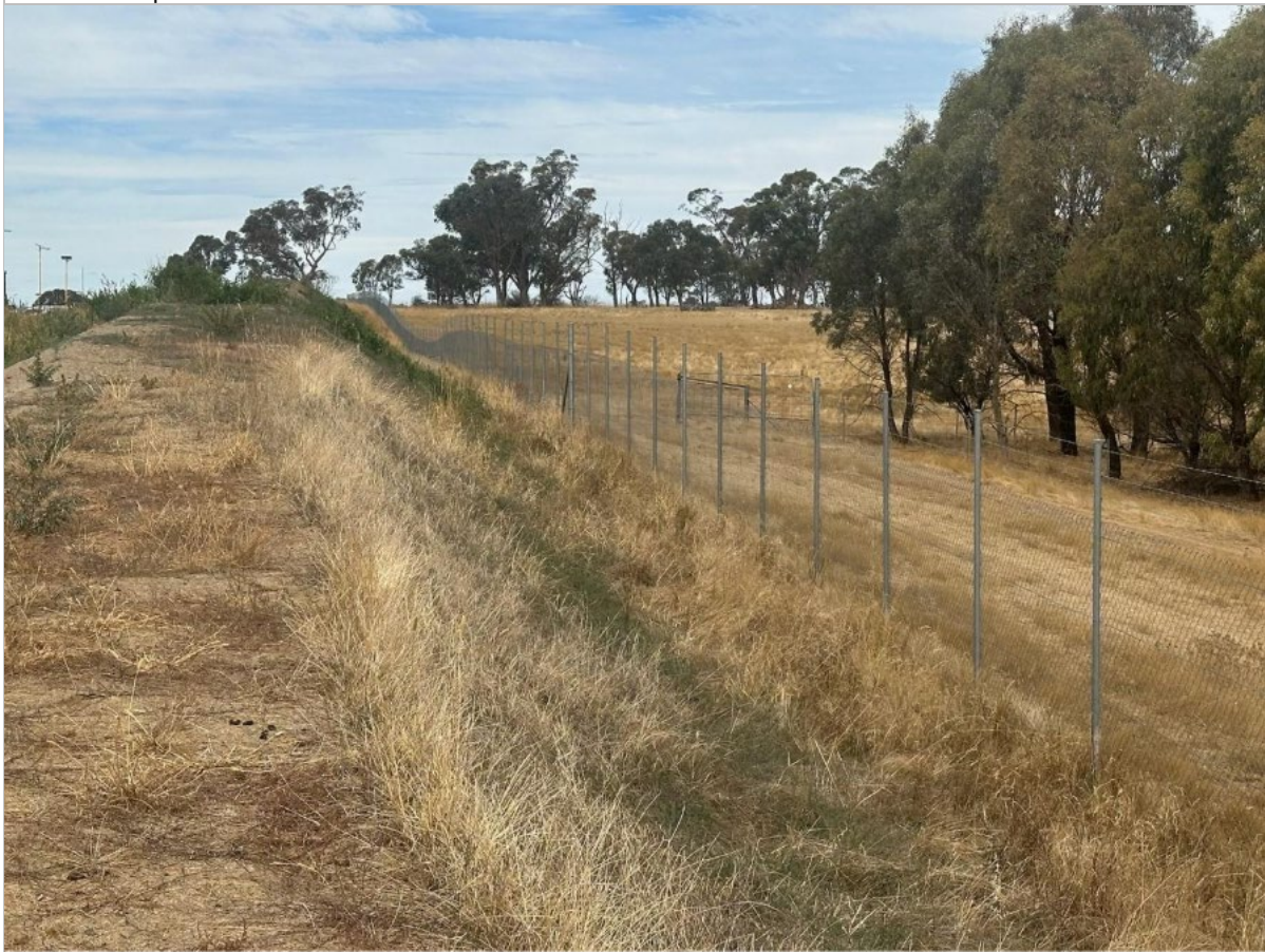
Photo 4: External bund and boundary fence
