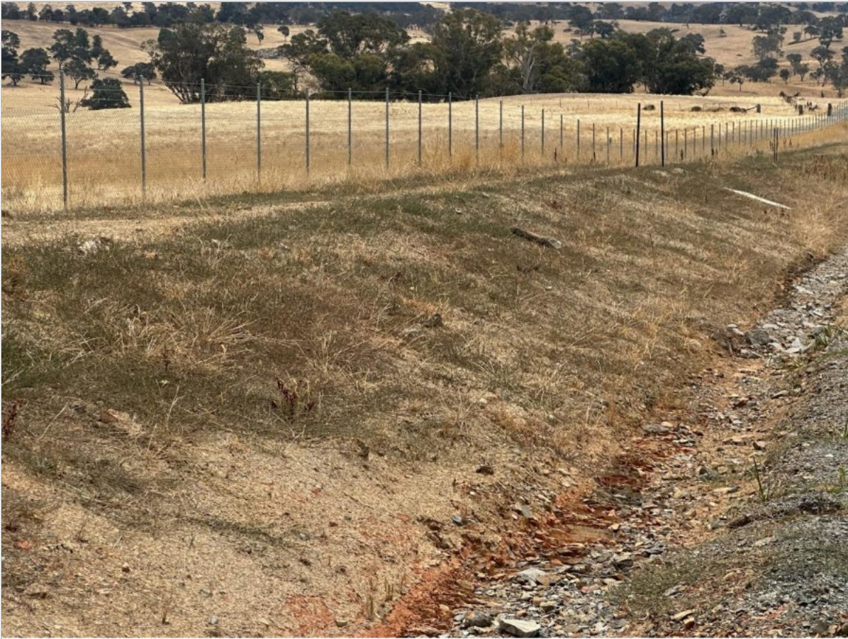
Photo 5: Stabilised batter and internal drain
