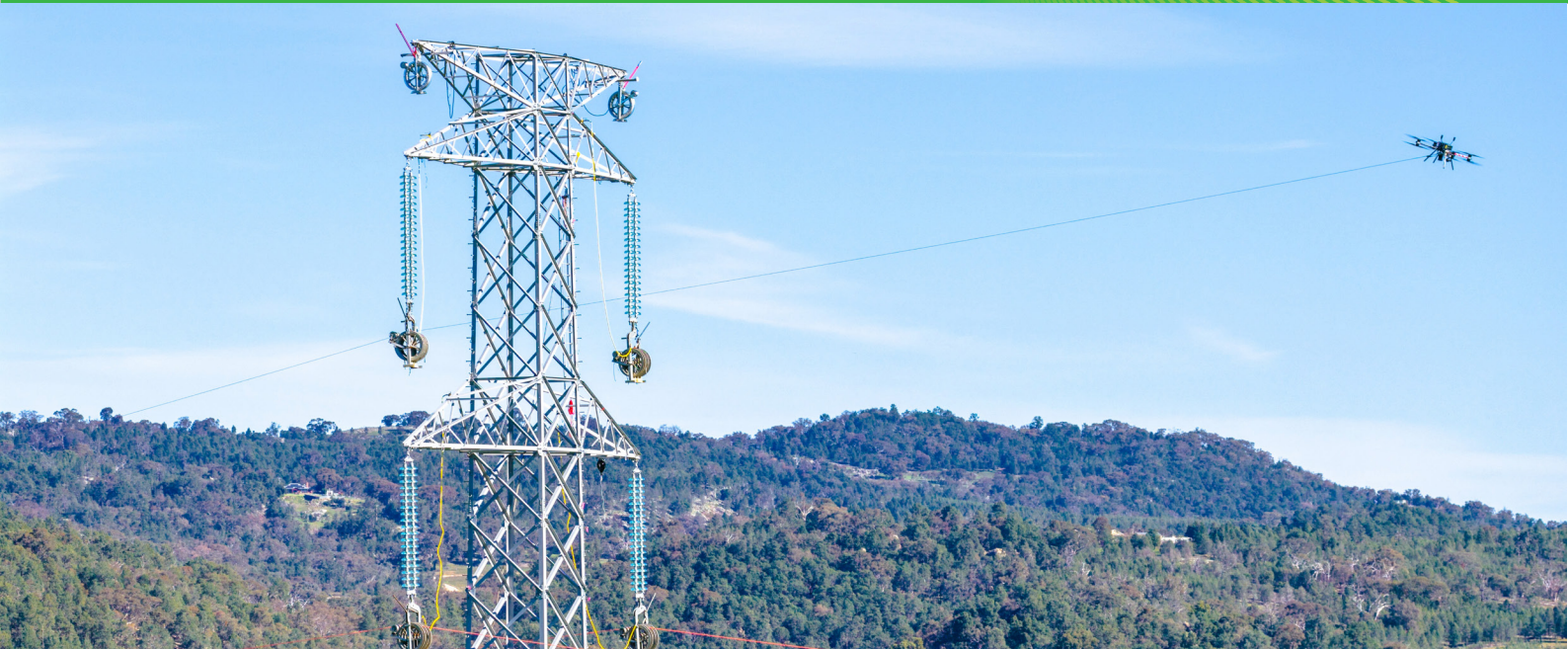
A specialised aerial stringing drone lifts a draw wire into place in preparation for conductor pulling on HumeLink West near Wagga Wagga.
