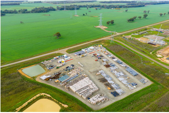
Tower steel and materials at Gregadoo ready for delivery to construction sites.
