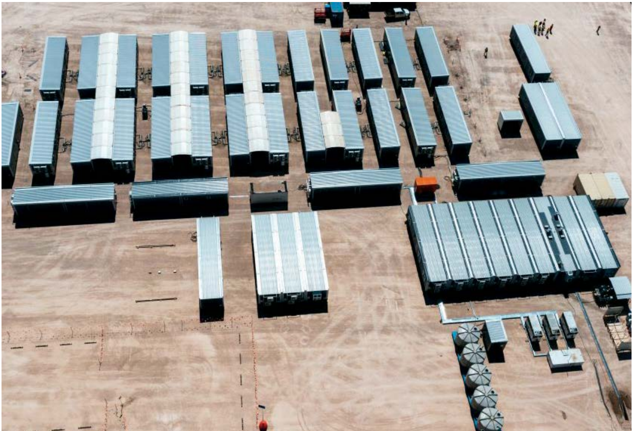
Pictured: Temporary construction compounds will be established at key locations.
