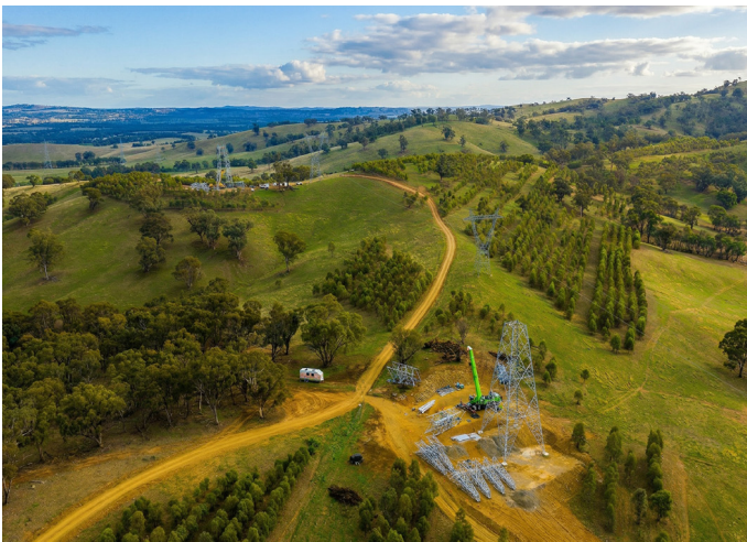
Another transmission tower nears completion on HumeLink West.
