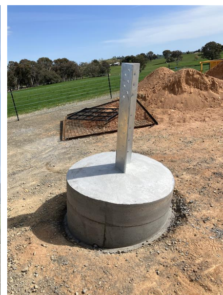
First tower stub concreted
