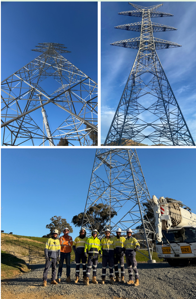
100th tower completed on HumeLink East, near Tumut.
