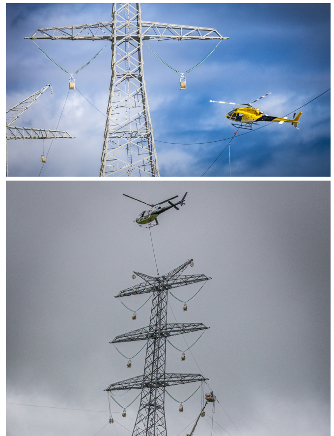
Helicopter stringing underway in Tumut and Adjungbilly.
