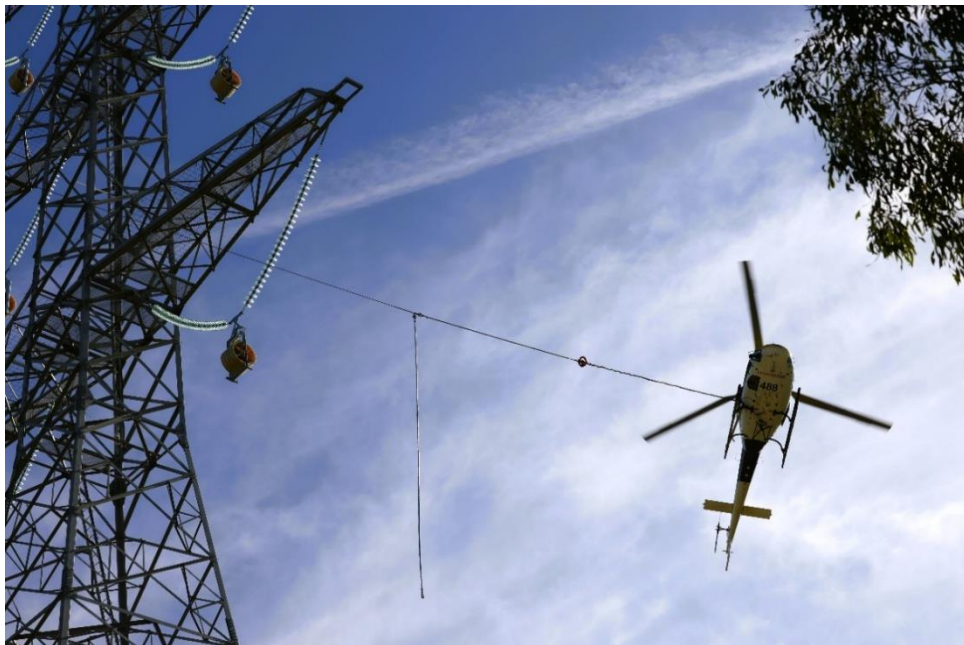
Helicopter stringing underway at Adjungbilly.
