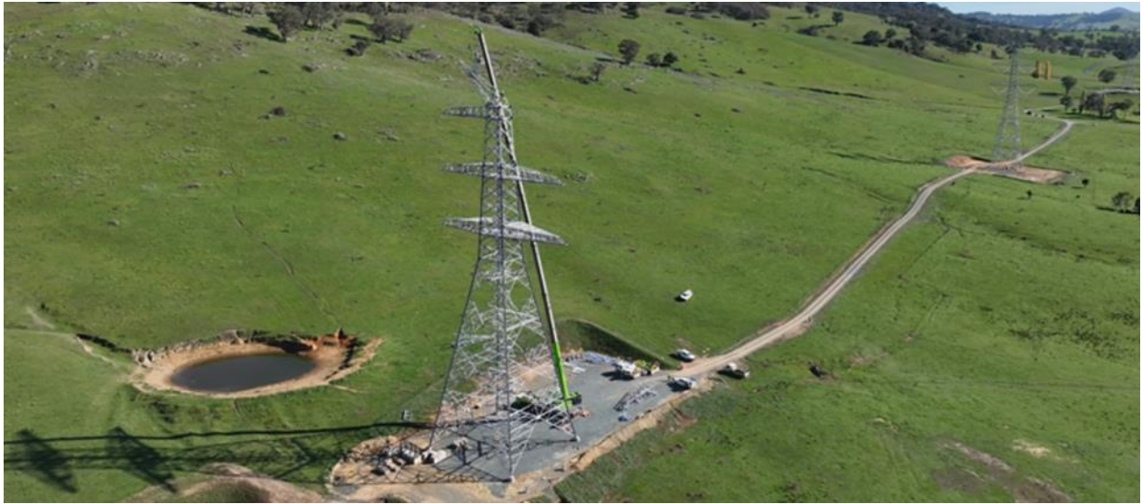
Completed interface tower (Tower 465) near Tumut.
