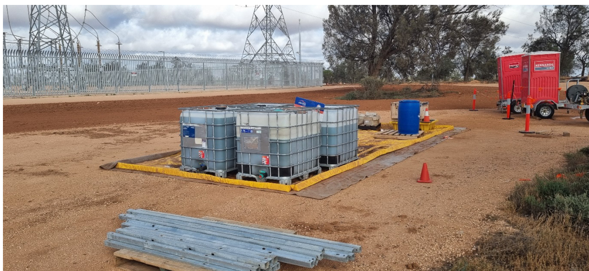
Photograph 3 – Temporary bunded hydrocarbon storage
