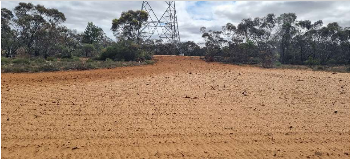
Photograph 5 – Typical Rehabilitated tower footprint
