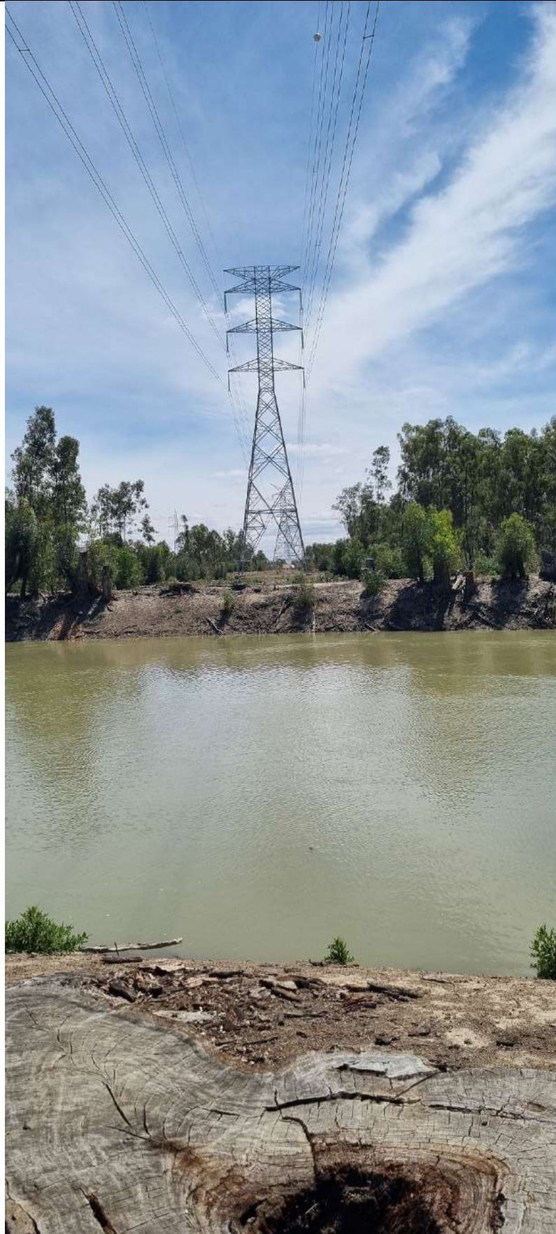
Photograph 8 – Murrumbidgee Crossing near Tower 513 (Line 2)
