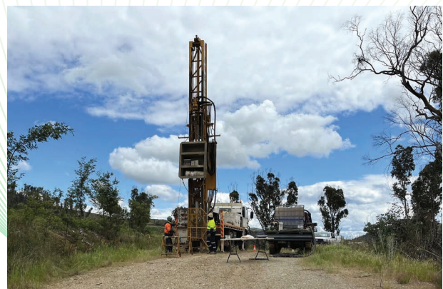
Image: truck mounted drill rig on site.
