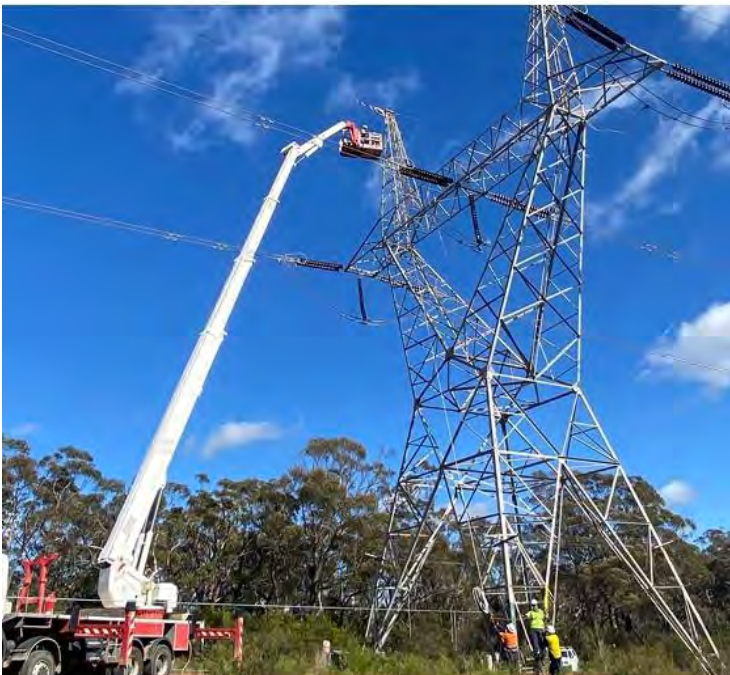
Figure 3.11. Typical transmission structure maintenance activity using an elevated work platform
