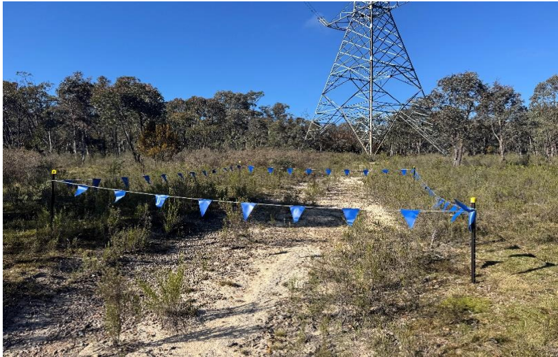
Figure 2 Flagging currently in place for pre-construction activities
