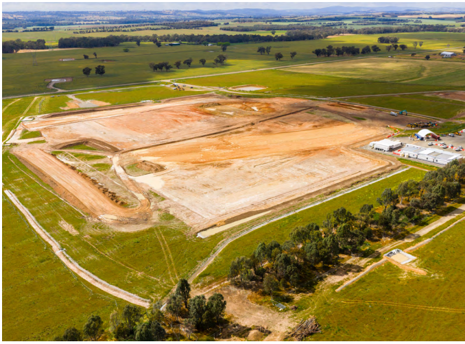
Bulk civil earthworks for the Gugaa Substation are nearing completion.
