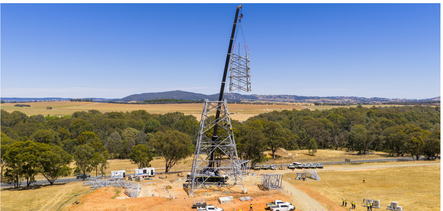
The first tower segments are lifted and bolted together during tower erection.
