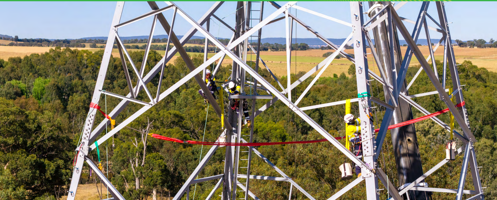
Workers in climbing safety harnesses help erect the first transmission tower on HumeLink West.
