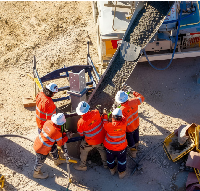
With the tower leg stub in place, the foundation pile is filled with concrete.
