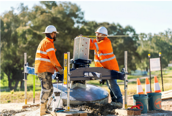
Each tower leg stub must exactly conform with the construction plan.
