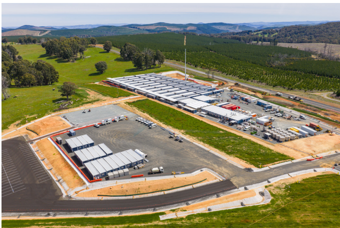
The Kunama worker accommodation facility near Batlow.
