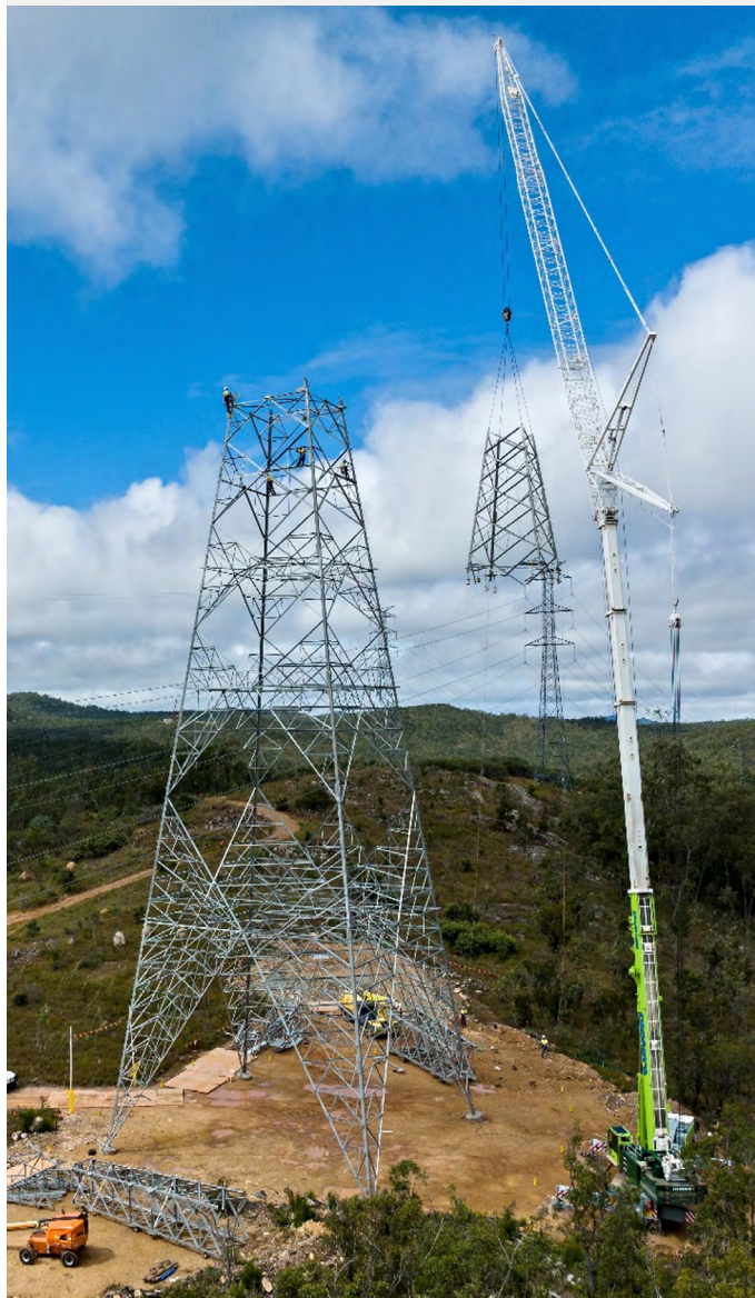
Construction of a similar transmission tower on an earlier project.
