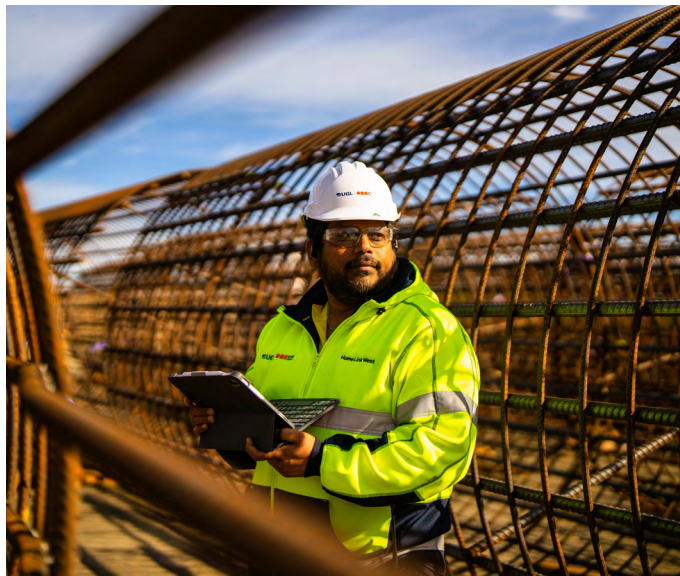
Logistics Manager, Ravindra Kolagani with pile cages for tower footings.
