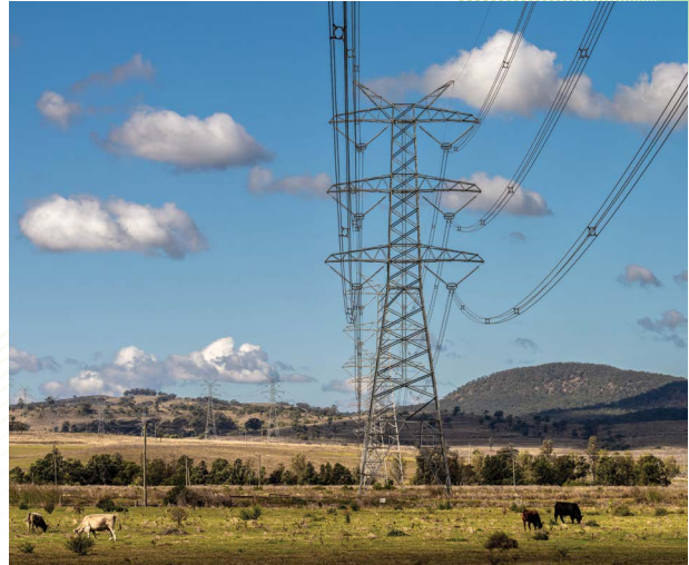
Pictured: Example of a 500 kV transmission tower.
