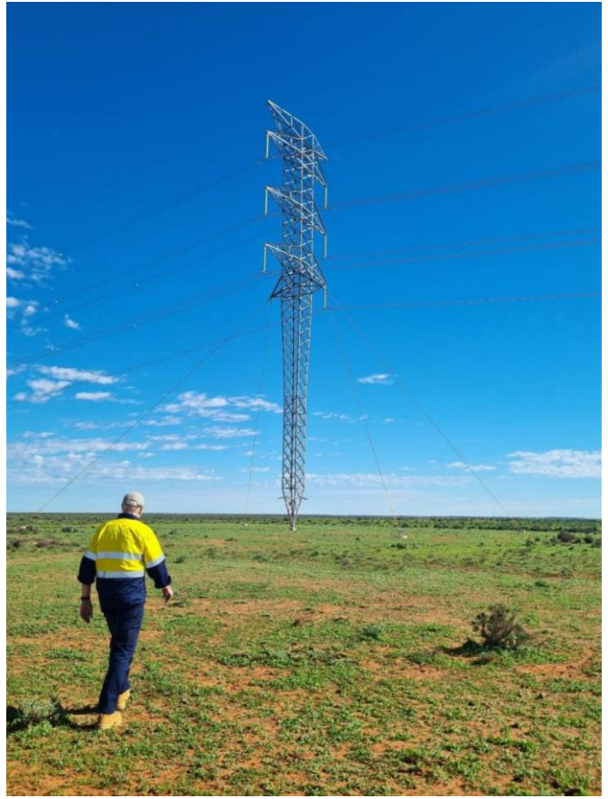
Photo 4: Guide Tower 222 showing groundcover regeneration.
