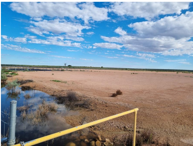
Photo 1: Former Camp 7 area, stabilised, no evidence of erosion, runoff controls and drainage in place.
