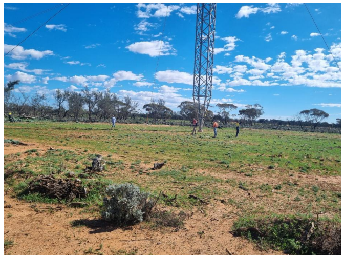
Photo 2: Guide Tower 252 showing groundcover regeneration.
