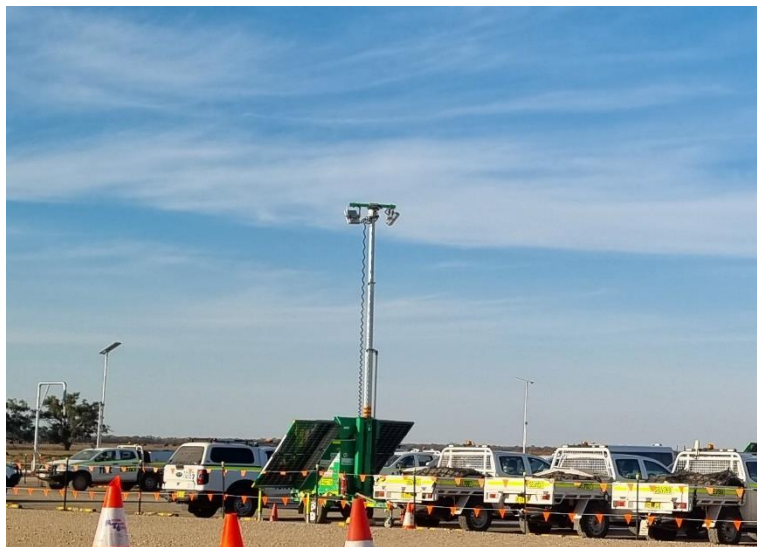
Photograph 6 – Camp 3 carpark lighting
