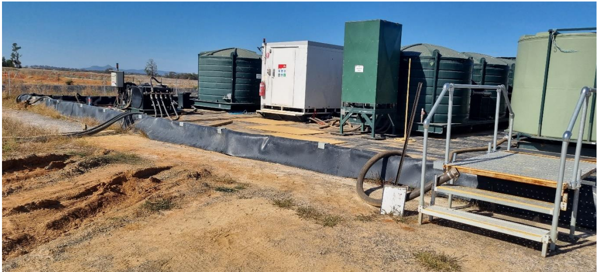
Photograph 10 – Camp 2 – bunding around water treatment plant.
