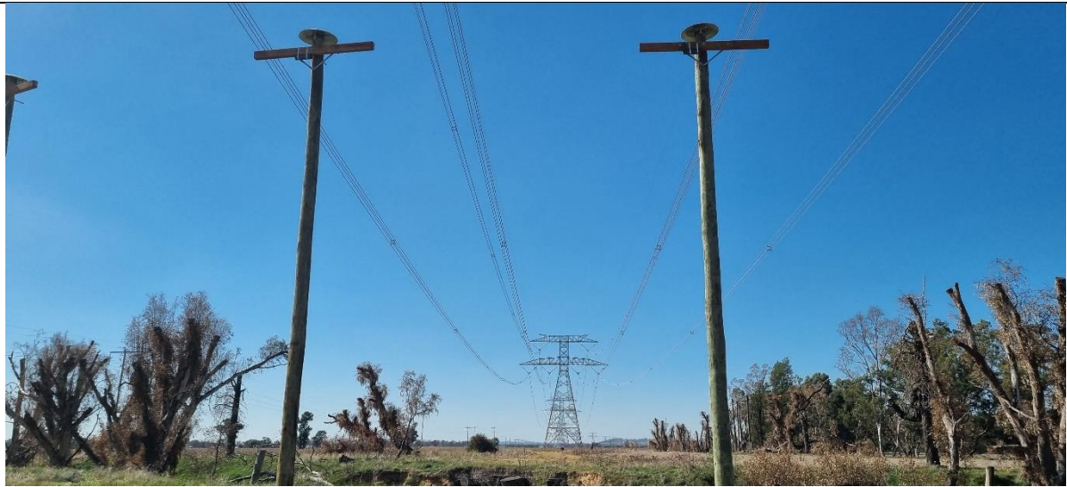
Photograph 12 – Glider poles installed between T71 and T72
