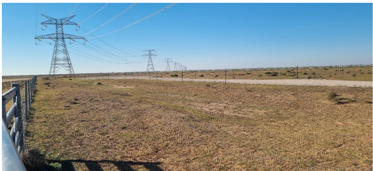
Photograph 7 – Rehabilitated broken winch site (T245) near Columbo Creek
