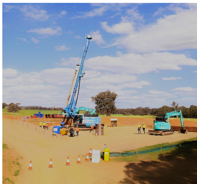
The first tower foundations have been drilled on HumeLink West.
