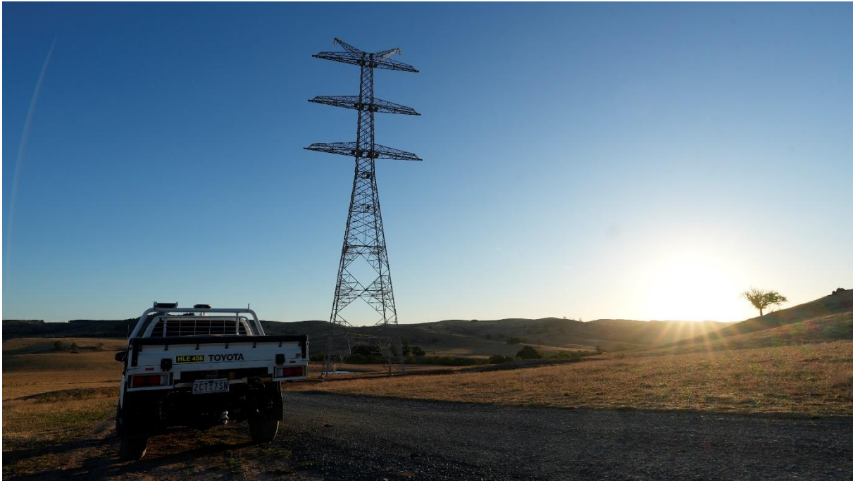
Tower 376, first completed tower near Adjungbilly, in January 2026.
