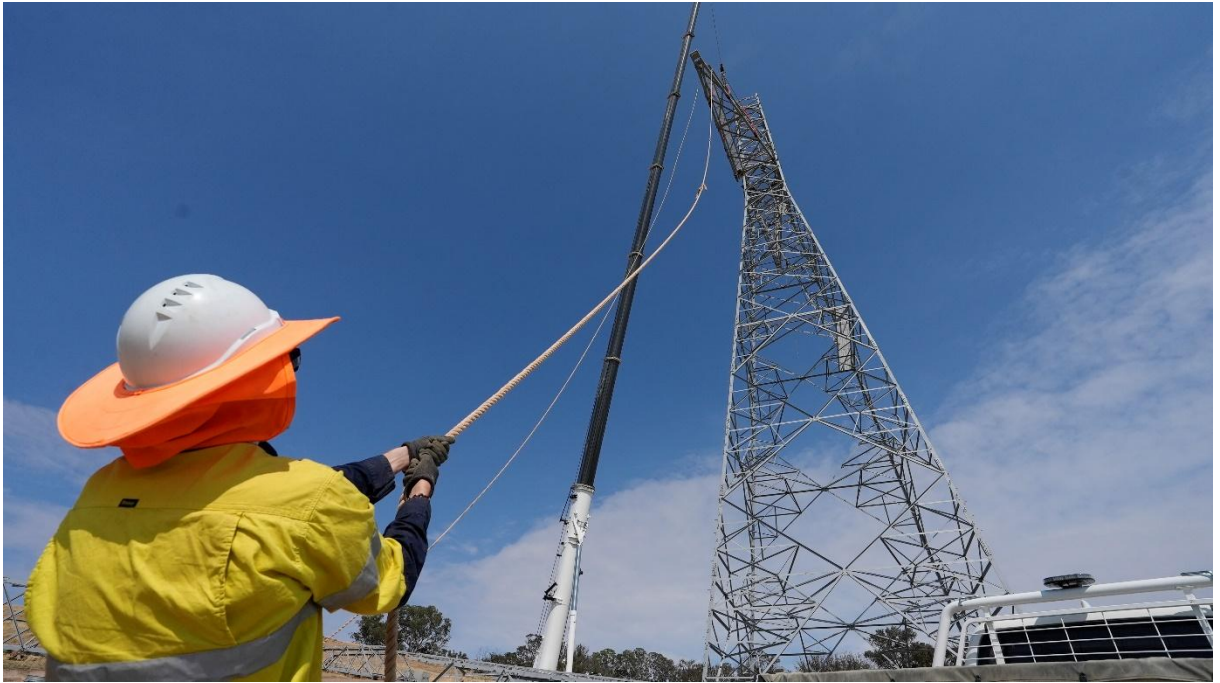
Tower construction underway in January 2026.
