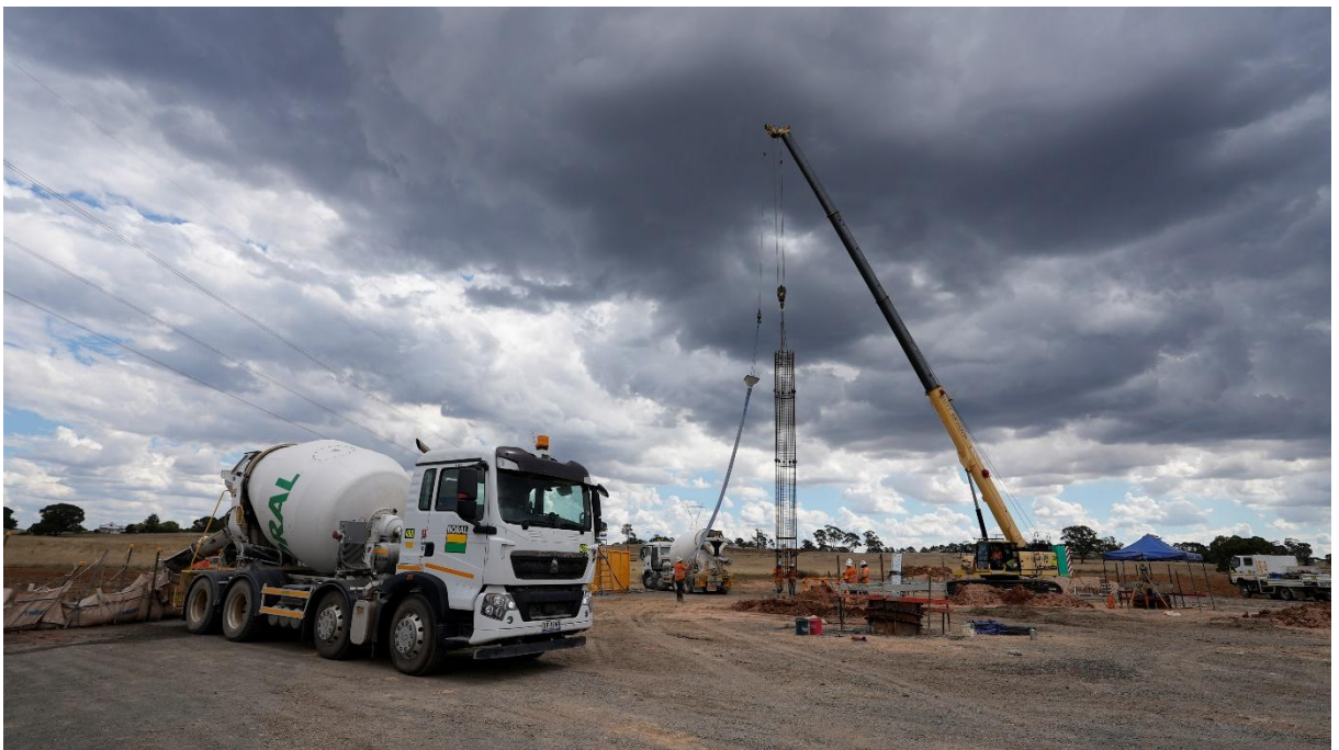
Piling works underway, with reinforcement cages being installed and concrete poured to establish the structural foundations.
