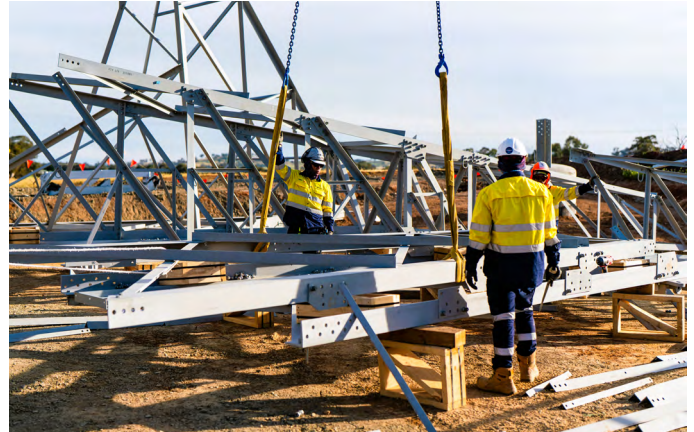
A transmission tower under assembly south-east of Wagga Wagga.
