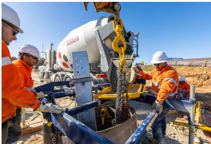
The first tower foundations have been poured on HumeLink West.
