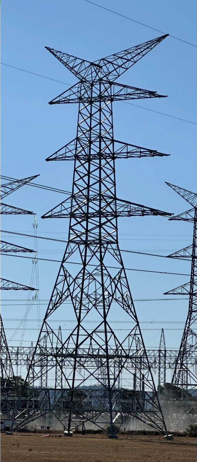
EnergyConnect 500kV tower adjacent to Wagga Substation
