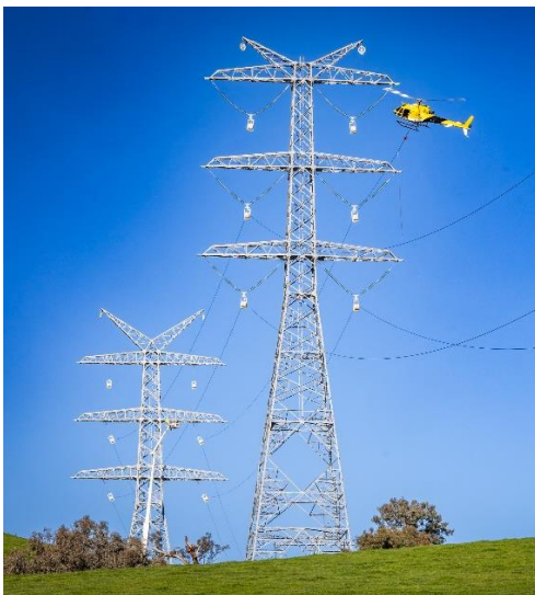
Examples of helicopter stringing on HumeLink East at Adjungbilly
