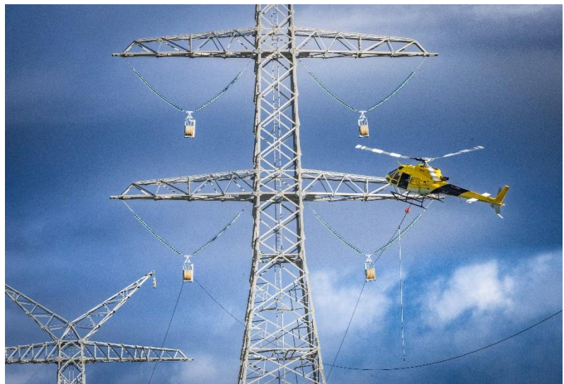
Examples of helicopter stringing on HumeLink East at Adjungbilly
