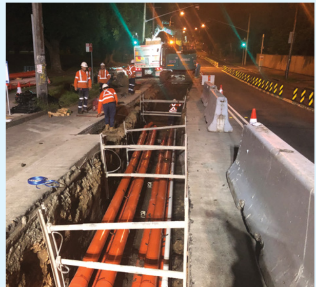
Night time trenching work on Old Canterbury Road, Ashfield
