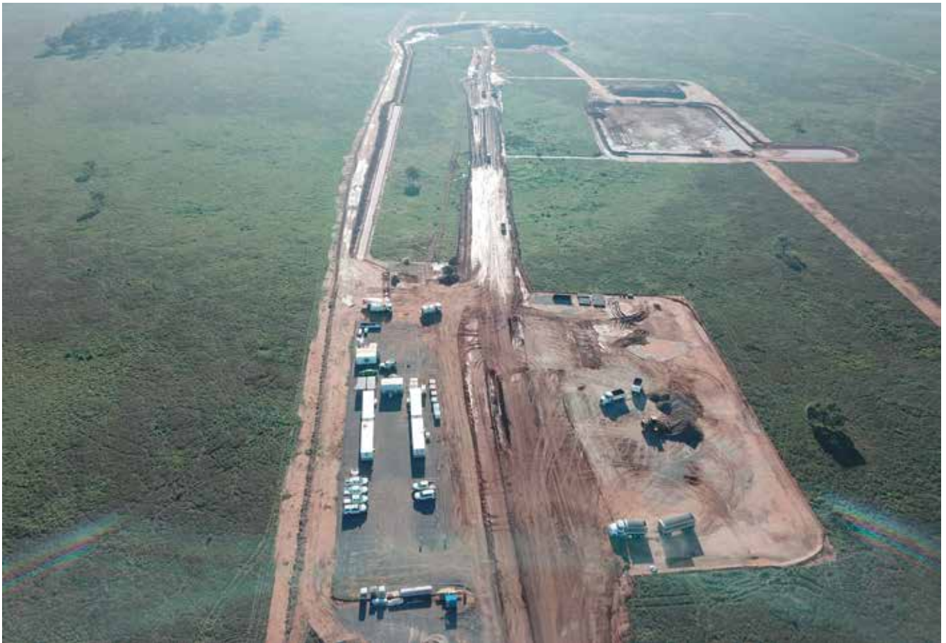
Image: Dinawan Substation Site
