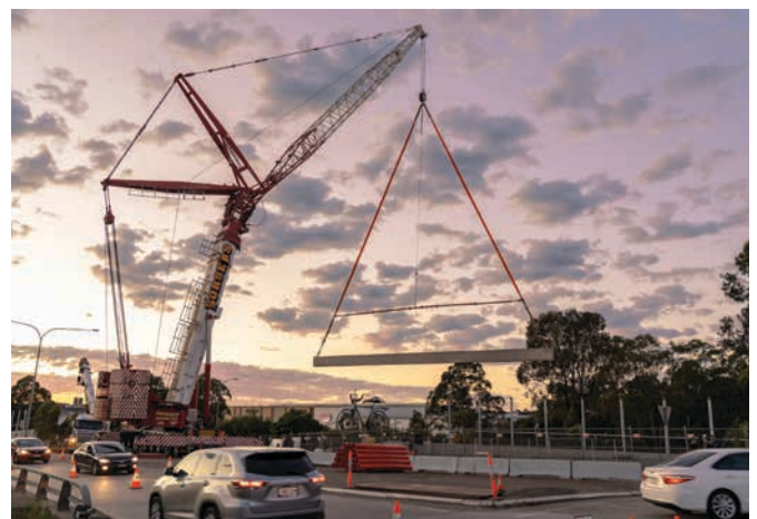
Muir Road cable bridge work during the October long weekend
