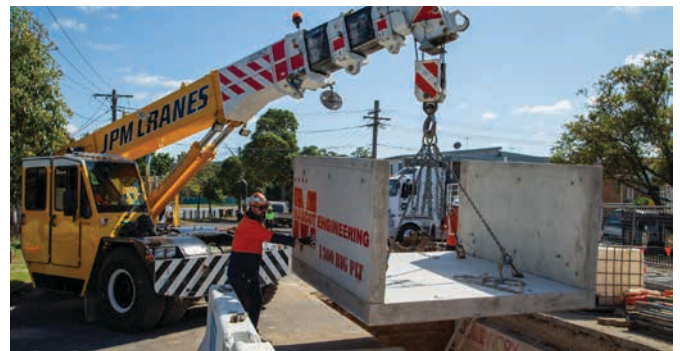
Joint bay construction at Hillcrest Avenue, Greenacre
