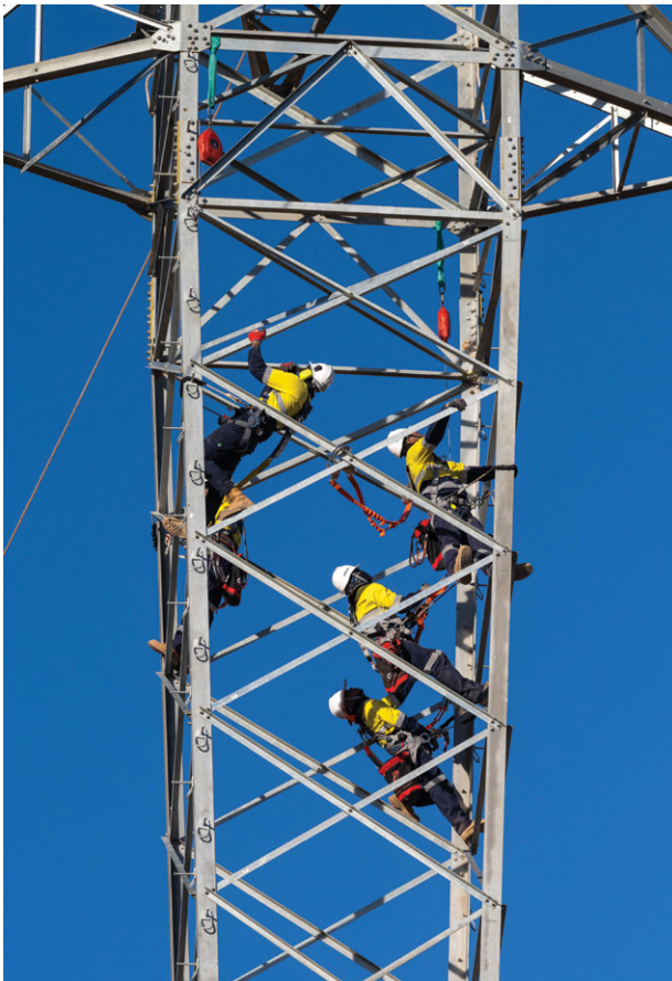
Pictured: A construction team assembling a 500 kV transmission tower onsite.
