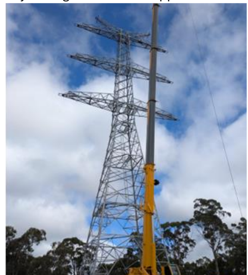
Bannaby substation works (left) and tower under construction (right)
