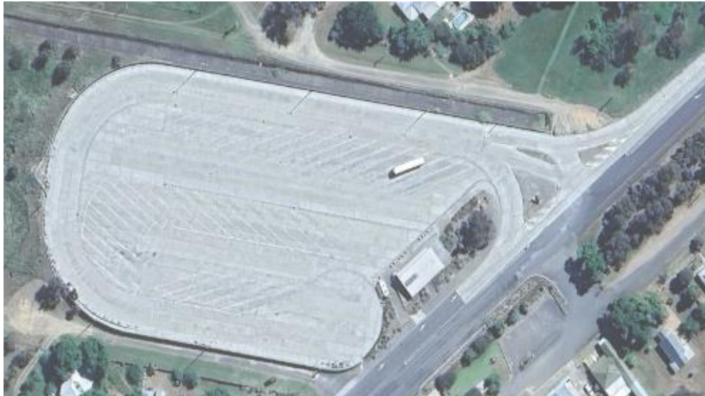
Figure 9: Tarcutta Truck Changeover Yard
