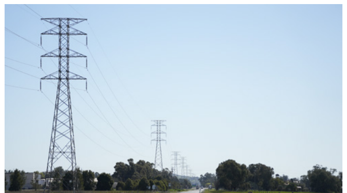
Image 2: Example of a 330 kV transmission line structure.
