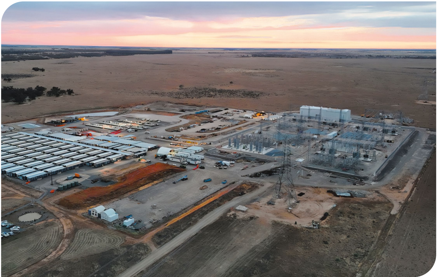
Figure: Dinawan substation during construction of EnergyConnect. The proposed 500 kV substation will be located to the right of the 330 kV substation.
