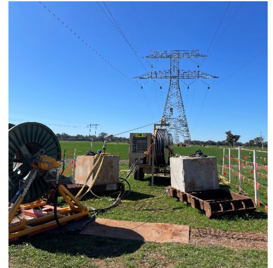
Image: Example of a break and winch site, Project Energy Connect
