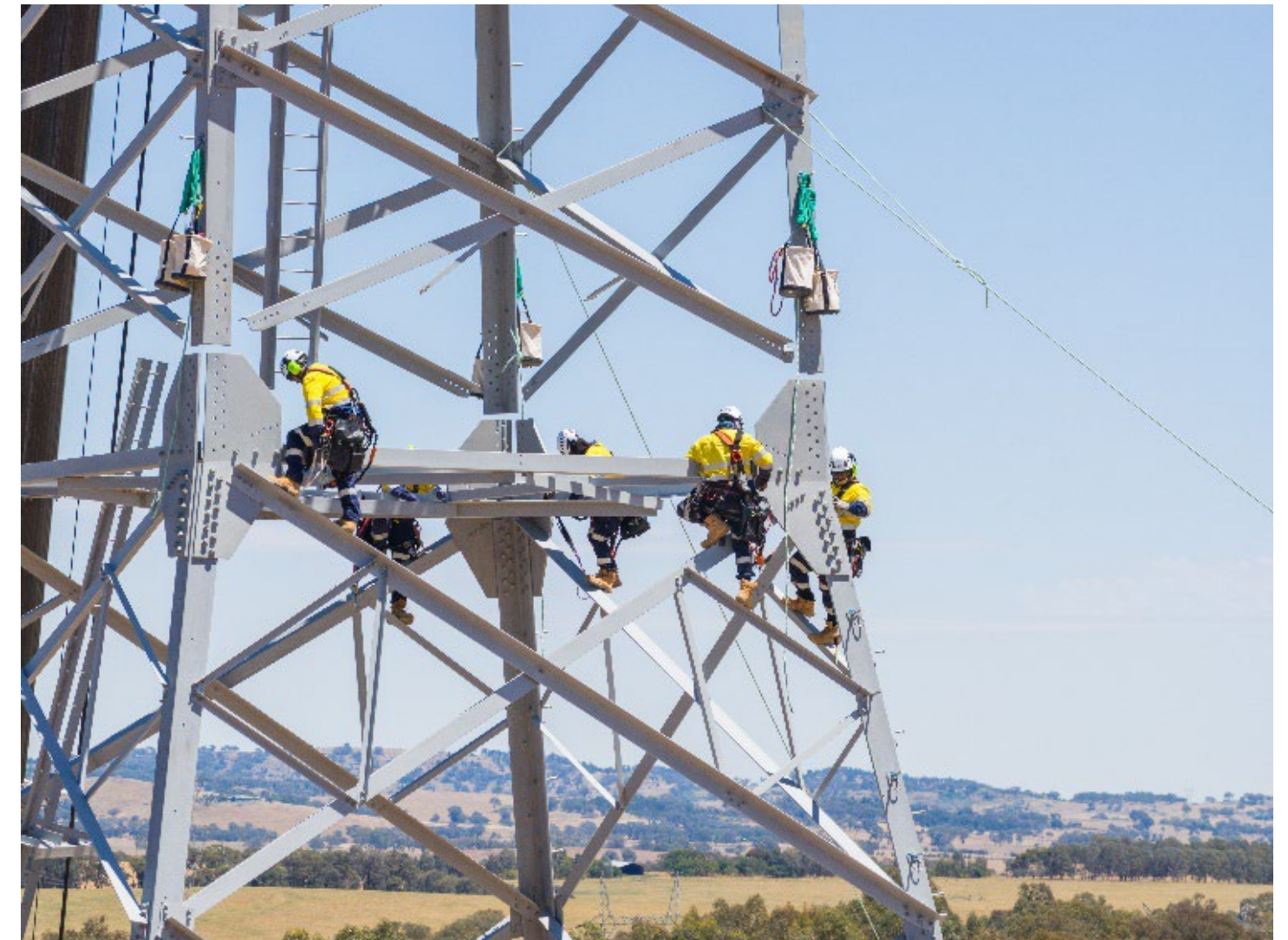
Image: HumeLink West 500kV tower construction
