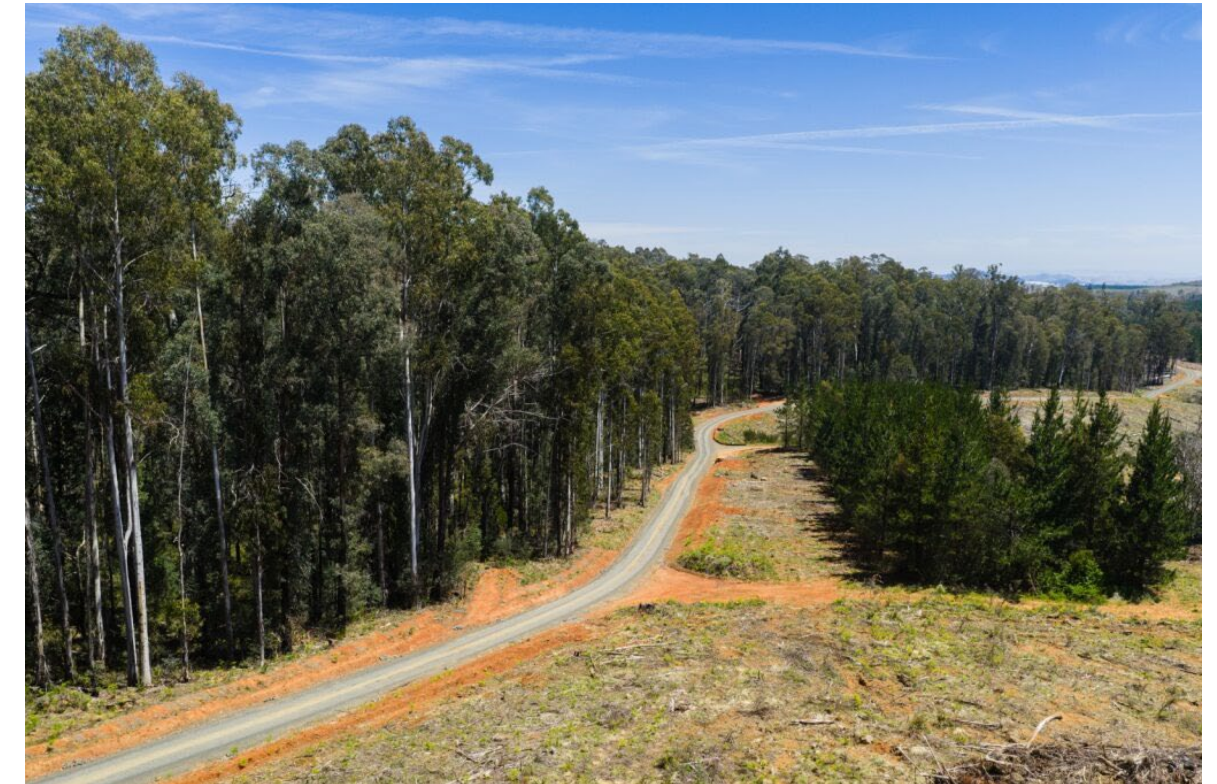
Image of an access track on the HumeLink project
