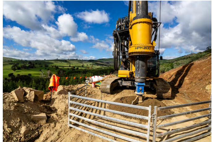
Rock fracturing makes it easier for drilling rigs to bore deep foundations.
