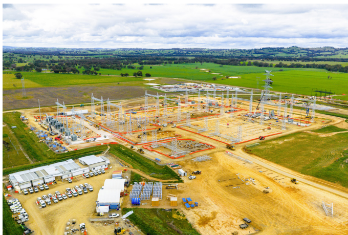
All of the overhead gantries have been installed at Gugaa Substation.
