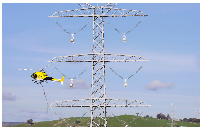
Helicopter stringing on HumeLink West is set to begin in October.
