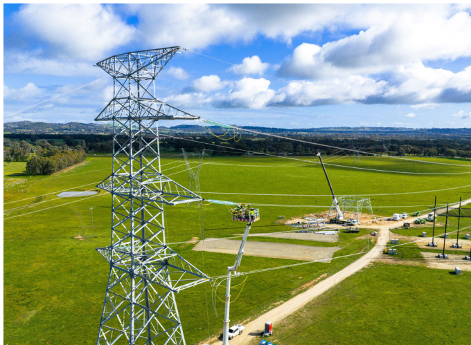
Workers installing conductor cables near Wagga Wagga.
