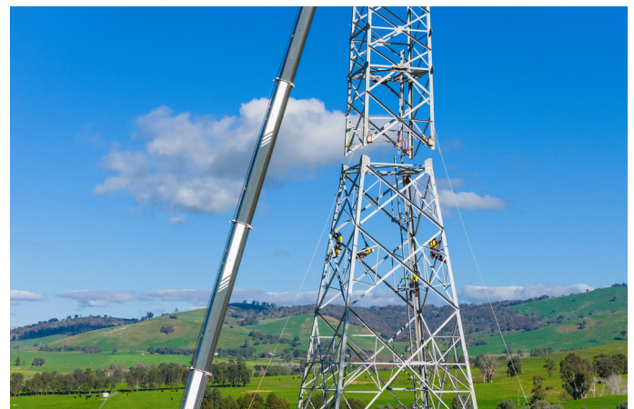
Workers at Ellerslie prepare to secure another tower segment into place.
