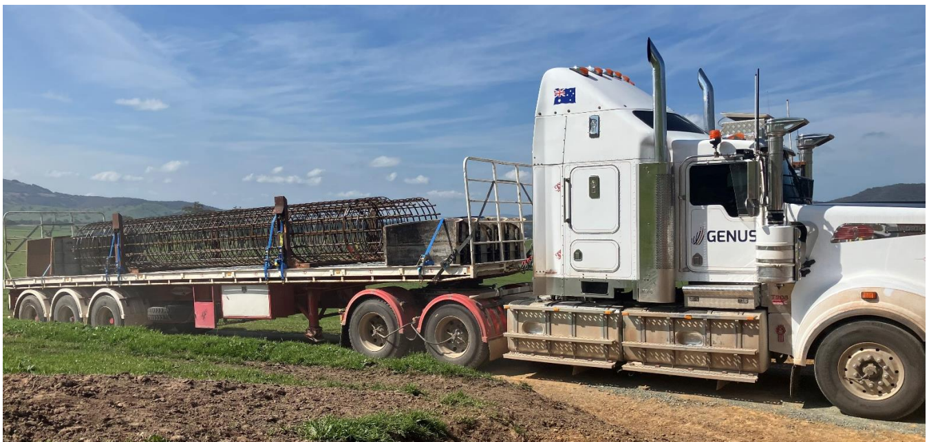
Foundation cages being delivered by truck near Tumut (September 2025)
