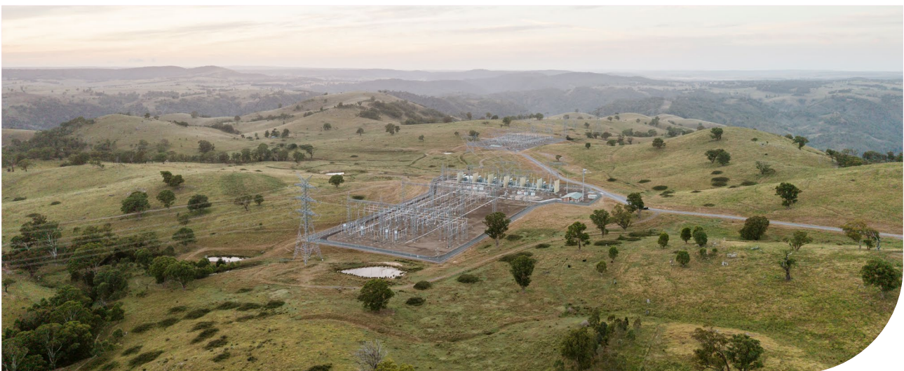
Bannaby 500/330 kV substation, NSW
