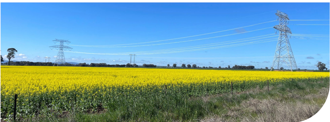
A 500 kV transmission line in South West NSW
